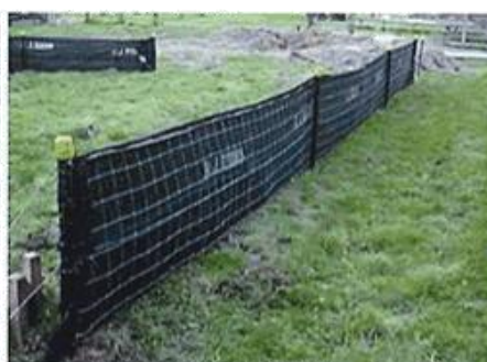
Figure 17 Example of a super silt fence. Retrieved from http://esccanterbury.co.nz/wp-content/uploads/2017/02/sc-super-silt-fence.jpg
