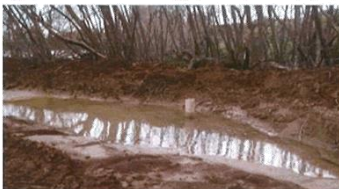
Figure 18 Example of a decanting earth bund. Retrieved from http://www.hortnz.co.nz/assets/Uploads/Auckland-Waikato-ES-Control-Guidelines-1-1.pdf
