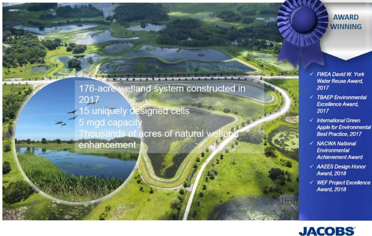
Figure 6 4G Infiltration Wetlands, Florida, USA
