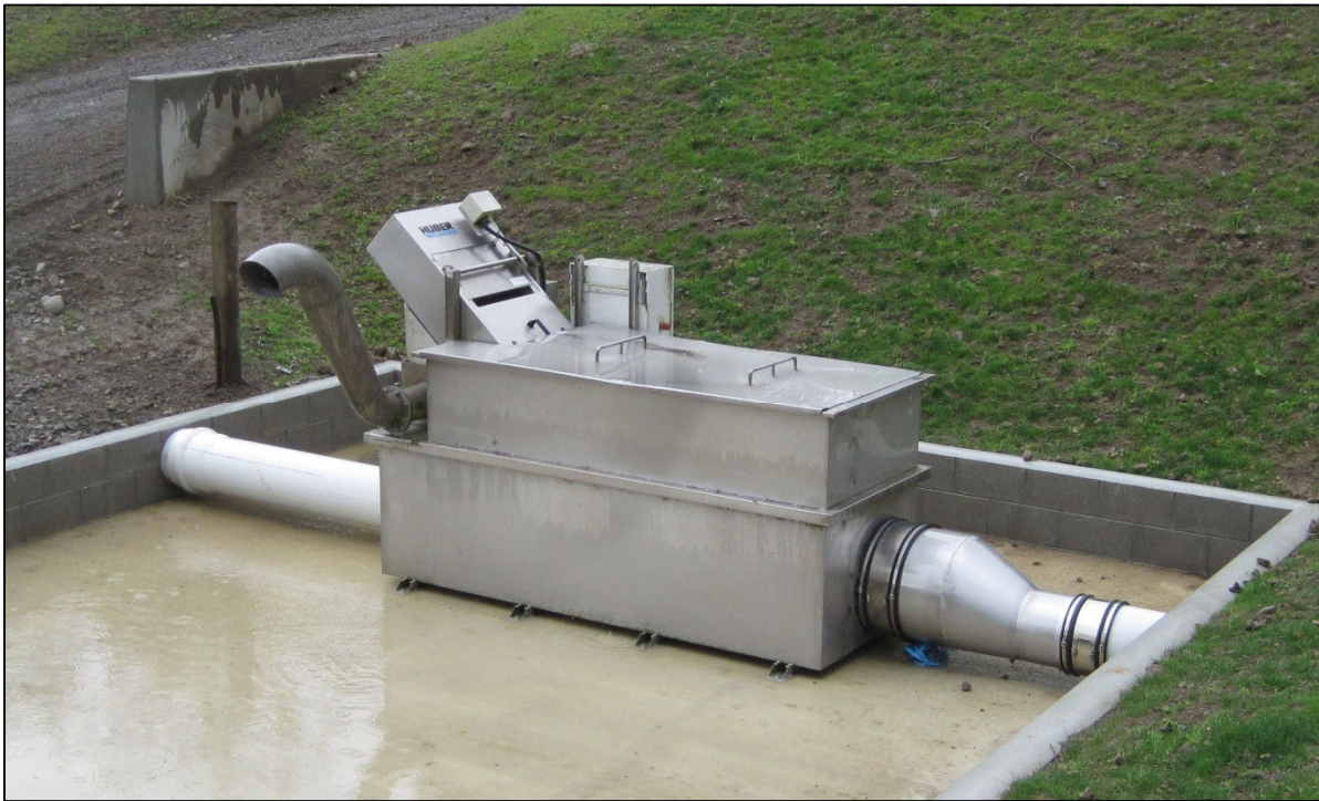
Figure 2: Step screen installed in 2014
