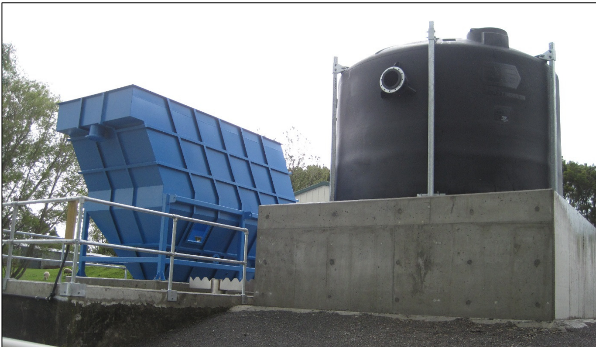
Figure 3: Installation of lamella plate clarifier (left) and contact tank (right) in progress
