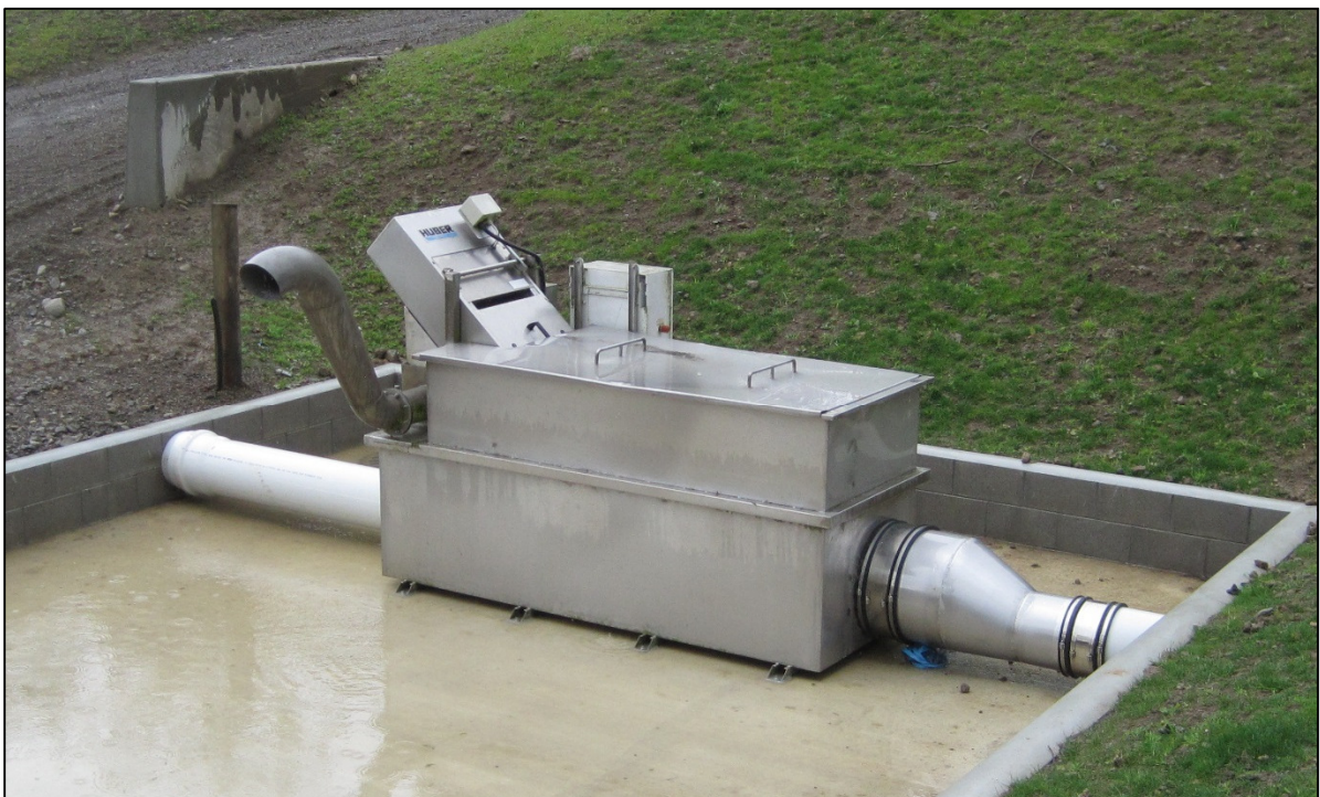
Figure 2: Step screen installed in 2014
