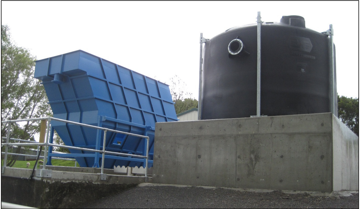
Figure 3: Installation of lamella plate clarifier (left) and contact tank (right) in progress (2014)
