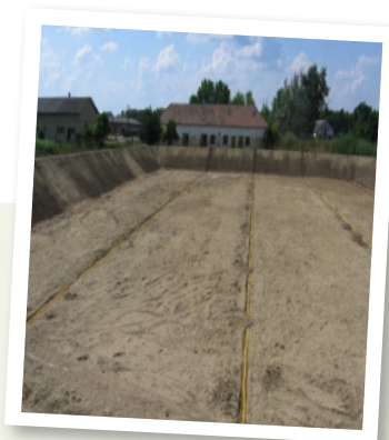
Grid pattern under floor drainage – prior to installation of liner
