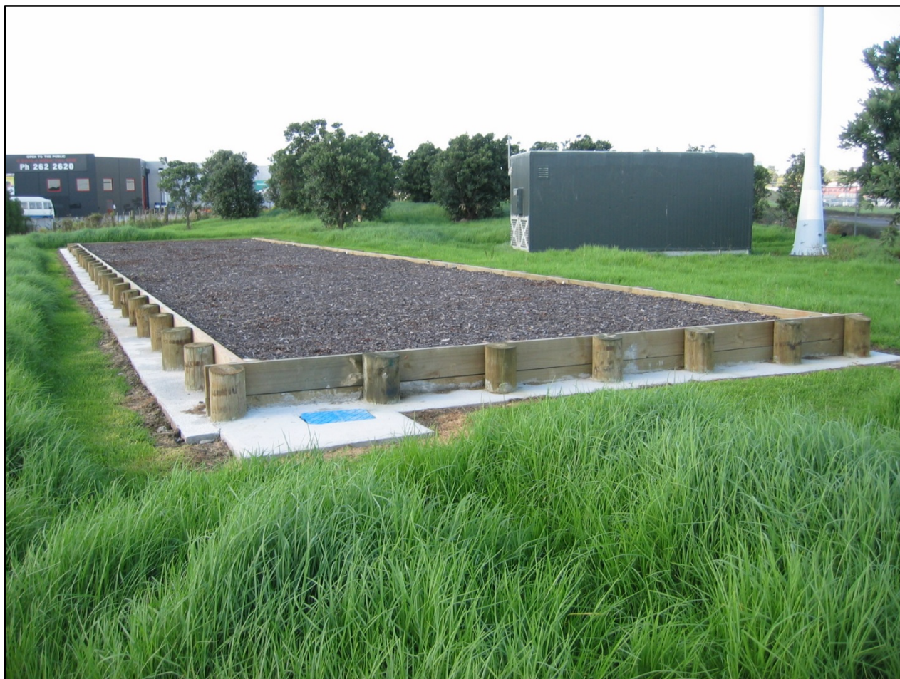
Figure 1–1: Photograph of a Biofilter with Bark Media
