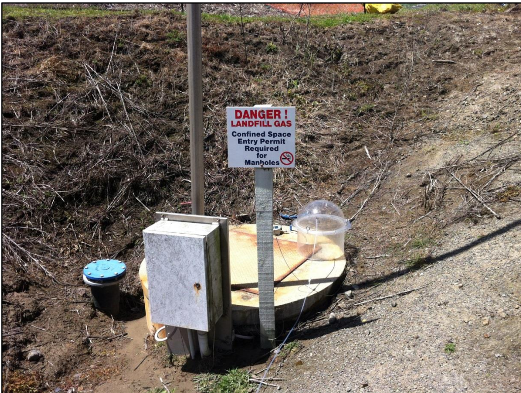
Figure C-4: Photo Looking East Showing Odour Monitoring at the Leachate Collection Manhole
