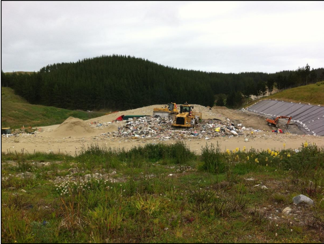
Figure C-1: Photo Looking West Showing the Stage 3 Active Landfill Area
