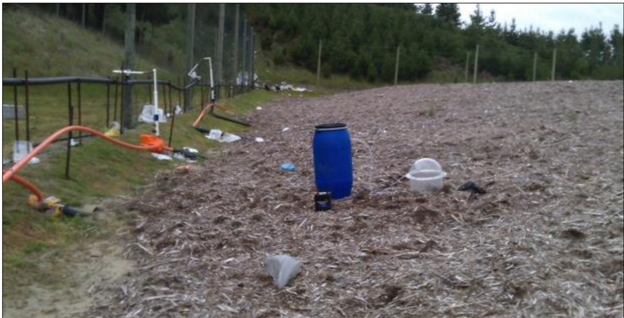
Figure 5.2 Sampling of the gas discharge identified during the walkover survey the preceding day.
