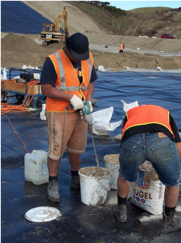
Photograph 9: HDPE liner welding Stage 1A (2004)
