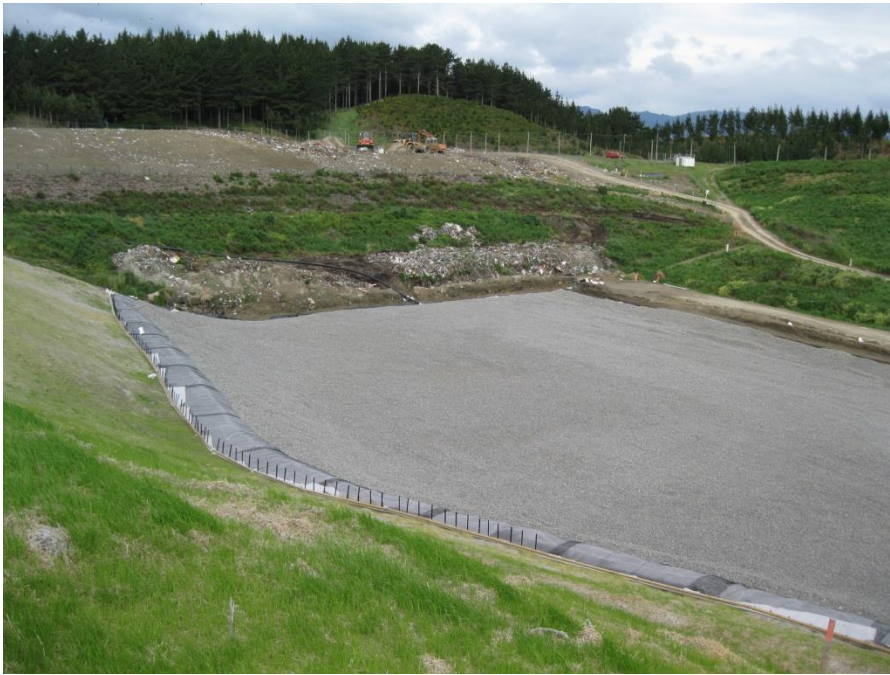
Photograph 5: Benching to sides of Stage 3A (2013)
