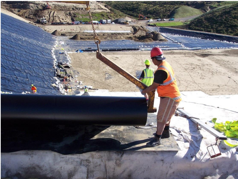
Photograph 7: GCL and HDPE liner construction Stage 1A (2004)
