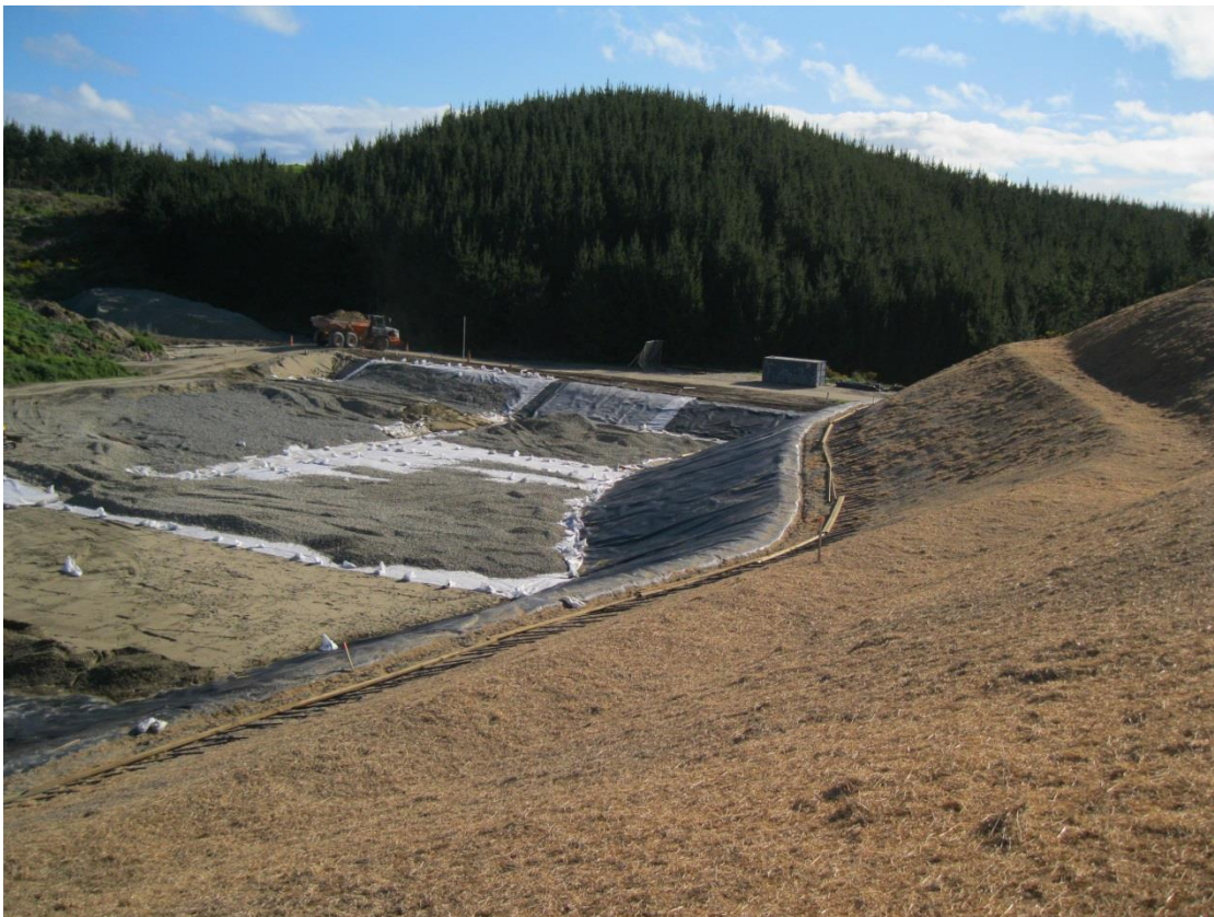
Photograph 5: Benching to sides of Stage 3A (2013)
