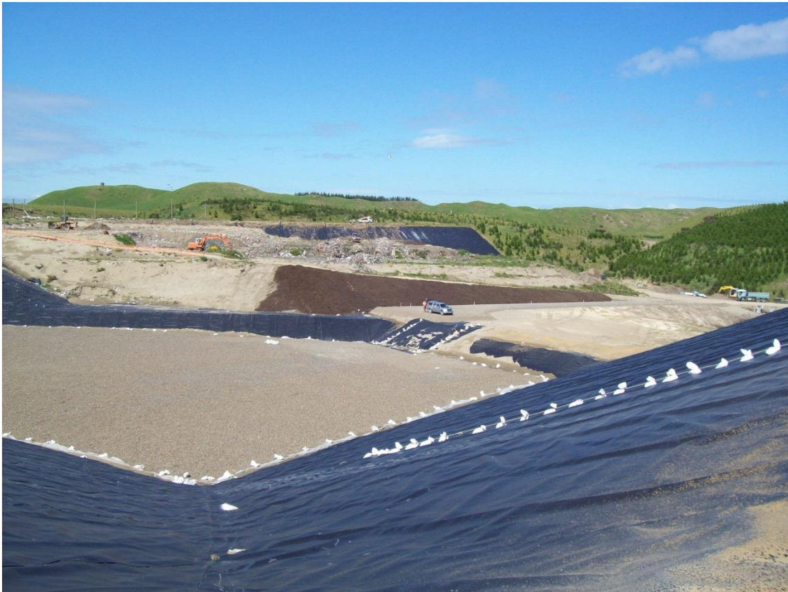
Photograph 17: Stage 2 liner completed
