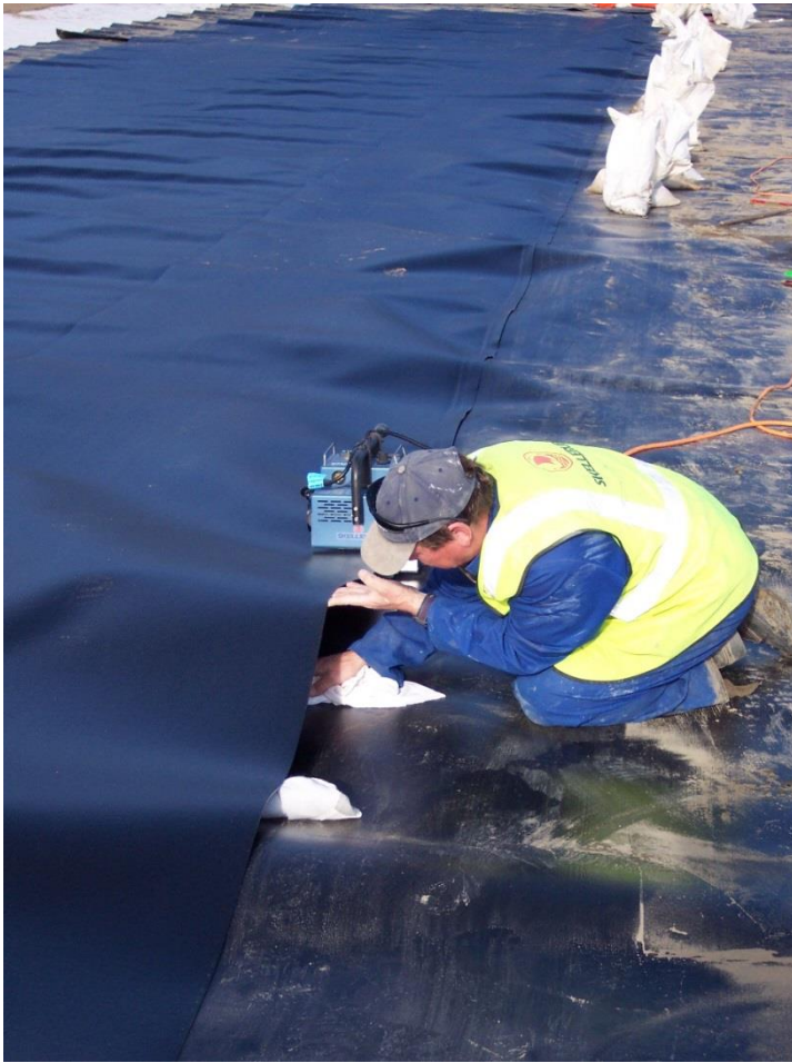
Photograph 7: GCL and HDPE liner construction Stage 1A (2004)
