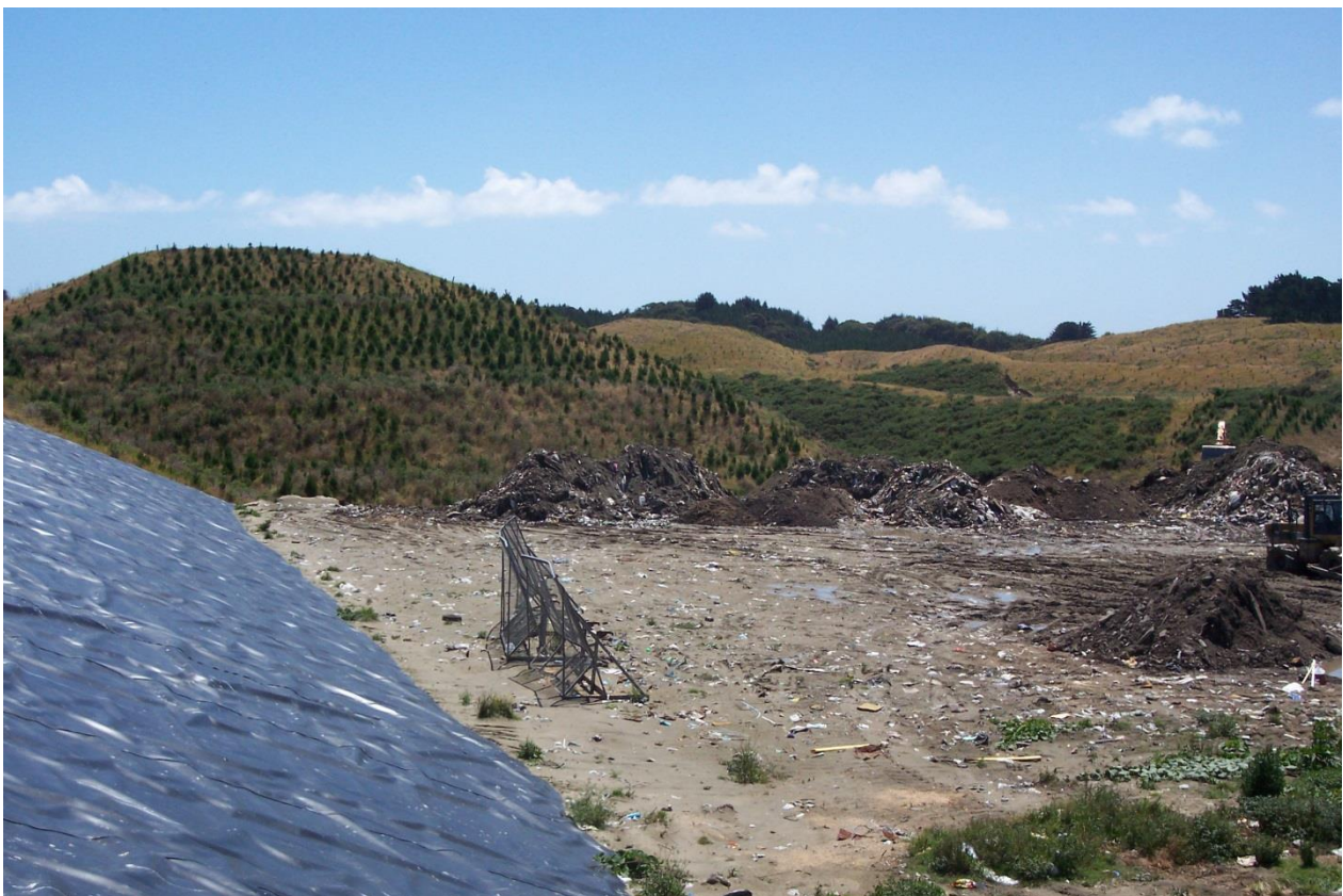
Photograph 2: Side liner of Stage 1A (2004 – 2005)
