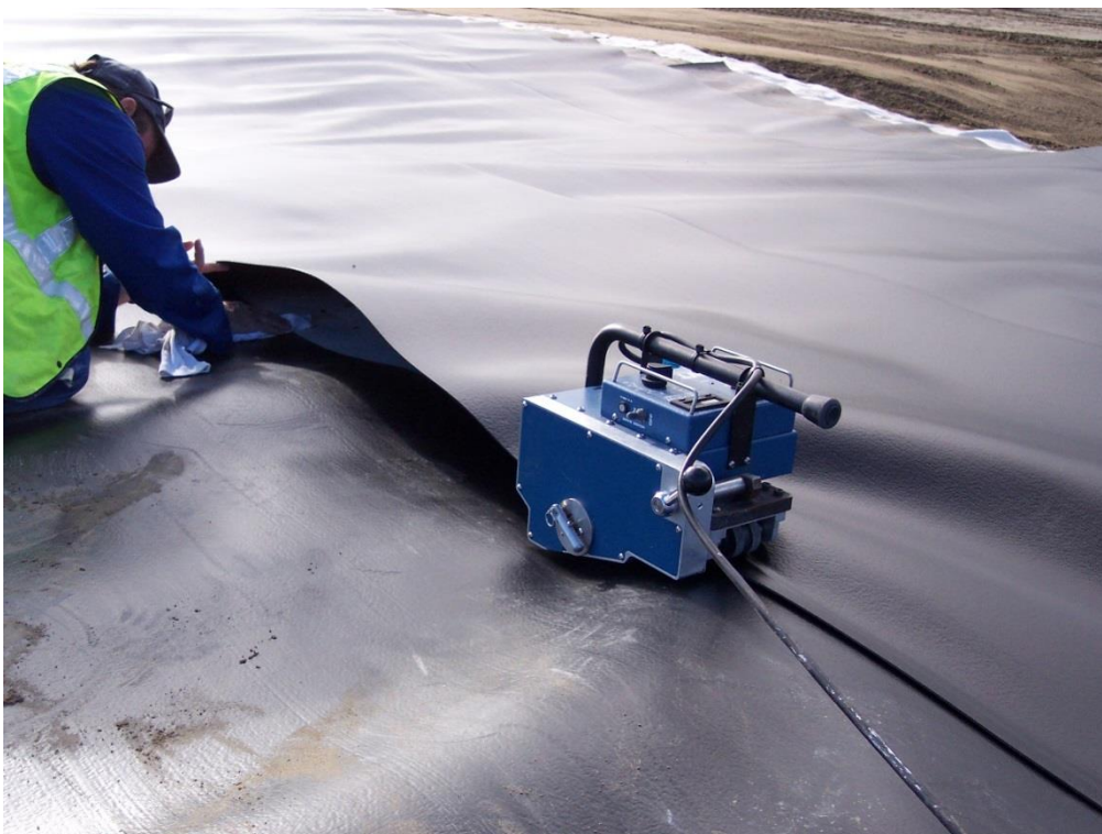
Photograph 9: HDPE liner welding Stage 1A (2004)
