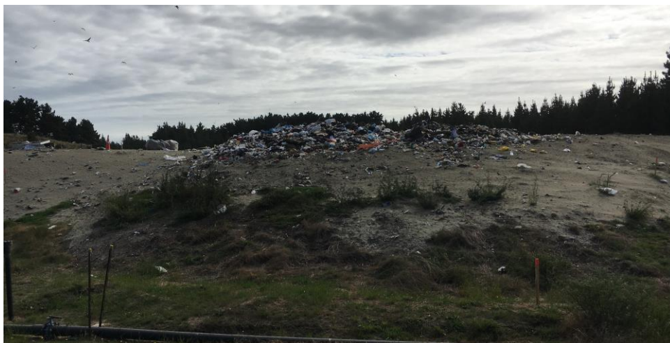
Figure 3 Stage 3 landfill area with sand and mulch intermediate cover (11 March, 2016)
