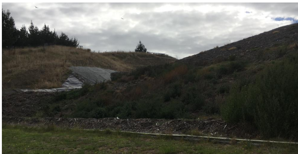
Figure 3 Stage 3 landfill area with sand and mulch intermediate cover (11 March, 2016)
