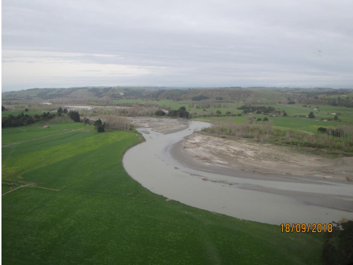
Out flanked bank protection
