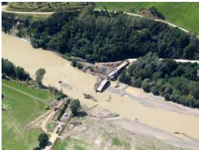
Figure 22. Loading of tree debris on bridge supports of the road bridge over the Pohangina River at Ashhurst contributed to its collapse during the flood. [GNS Photo: GH 1189].
