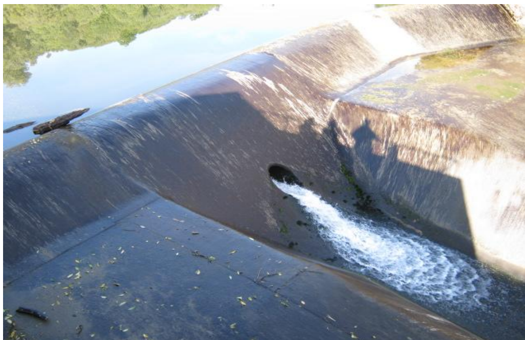
Figure 4: The 25l/s Outlet from the Lower Dam
