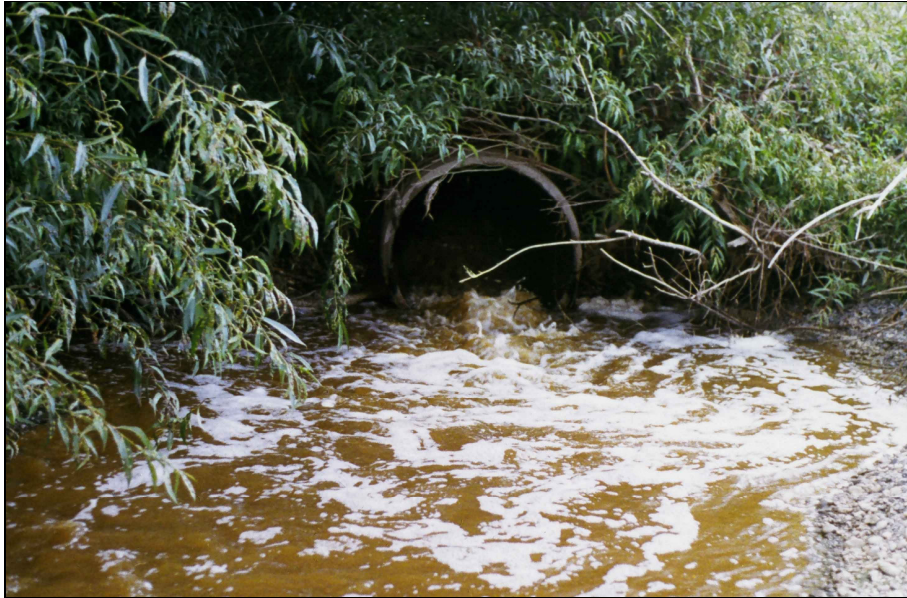
Figure 1. Feilding sewage treatment plant outfall (circa 1980)
