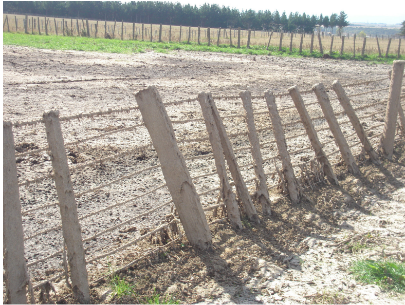
Figure 1. Effluent build-up on a fence and surrounding pasture resulting from a broken effluent irrigator. The irrigator had been broken for many days.
