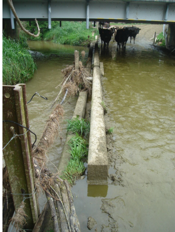
Figure 4. Stock accessway beneath a road bridge, located alongside a stream. Stock effluent, which naturally accumulates on the low part of the race, is flowing freely into the stream.
