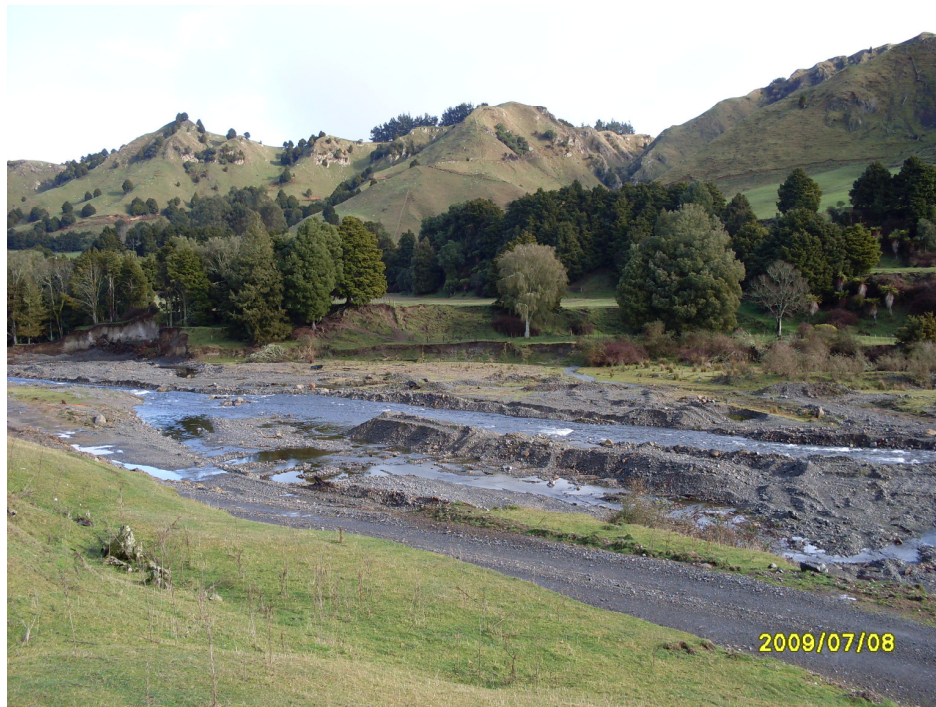
Figure 7. Ground-based view of the illegal channel works on the Taringamotu River (taken earlier than the aerial views above). This image is taken from the approximate position of the front-end loader in the aerial views above.
