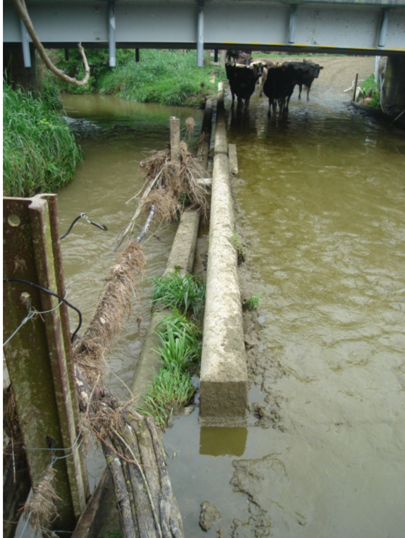
Poorly located and inadequately managed underpass. Subsequently, effluent discharged from underpass into a tributary of the Manawatu River.
