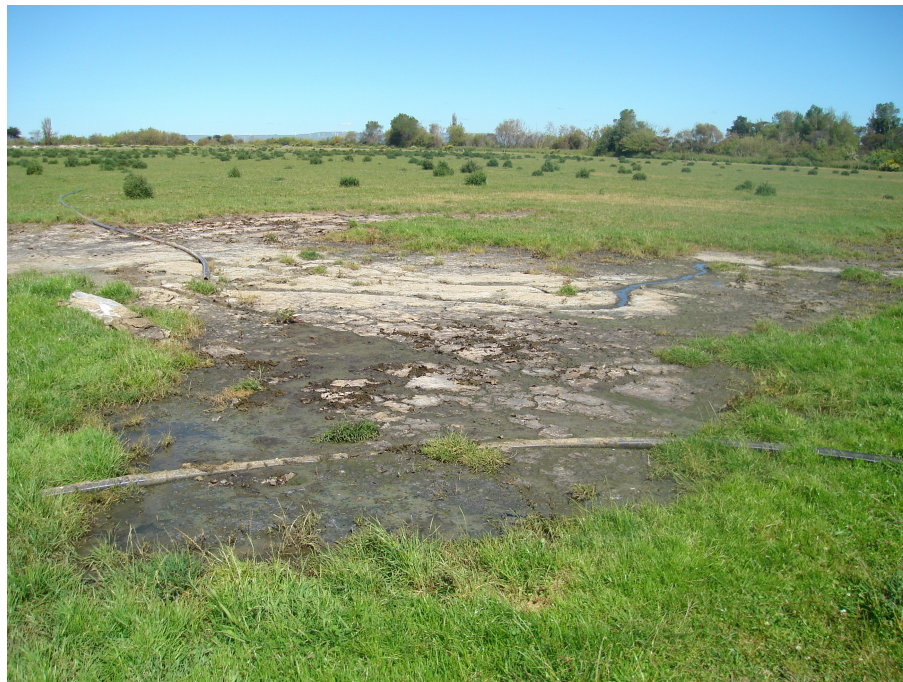
Further photos of ponding as detailed above. Solids indicated that the discharge had been occurring for some time.
