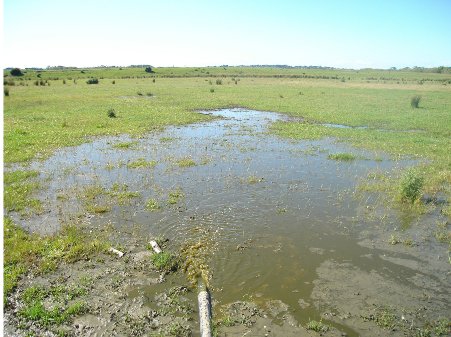
Significant ponding from a naked end pipe causing the type of effluent management that resulted in a prosecution under section 151(b) of the Resource Management Act 1991
