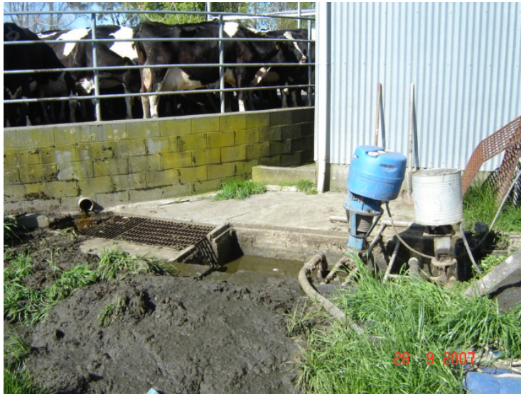
Undersized sump showing clear evidence of overflow. This was the only storage available for the dairy shed effluent on this farm.
