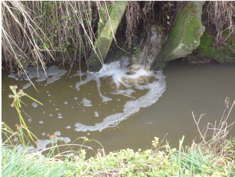
Discharge from tile drain due to effluent been discharged onto land at too higher rate.
