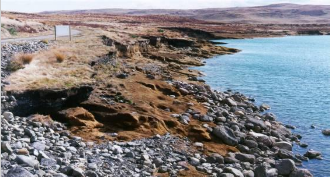
Shoreline erosion near Moawhango Dam.
