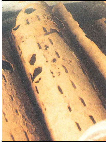
Figure 15. Example of erosion causing damage to screen and eventual failure of the well as a result of incrustation and corrosion due to iron precipitation and bacteria growth (Photo from: Driscoll, 1986) 25 .
