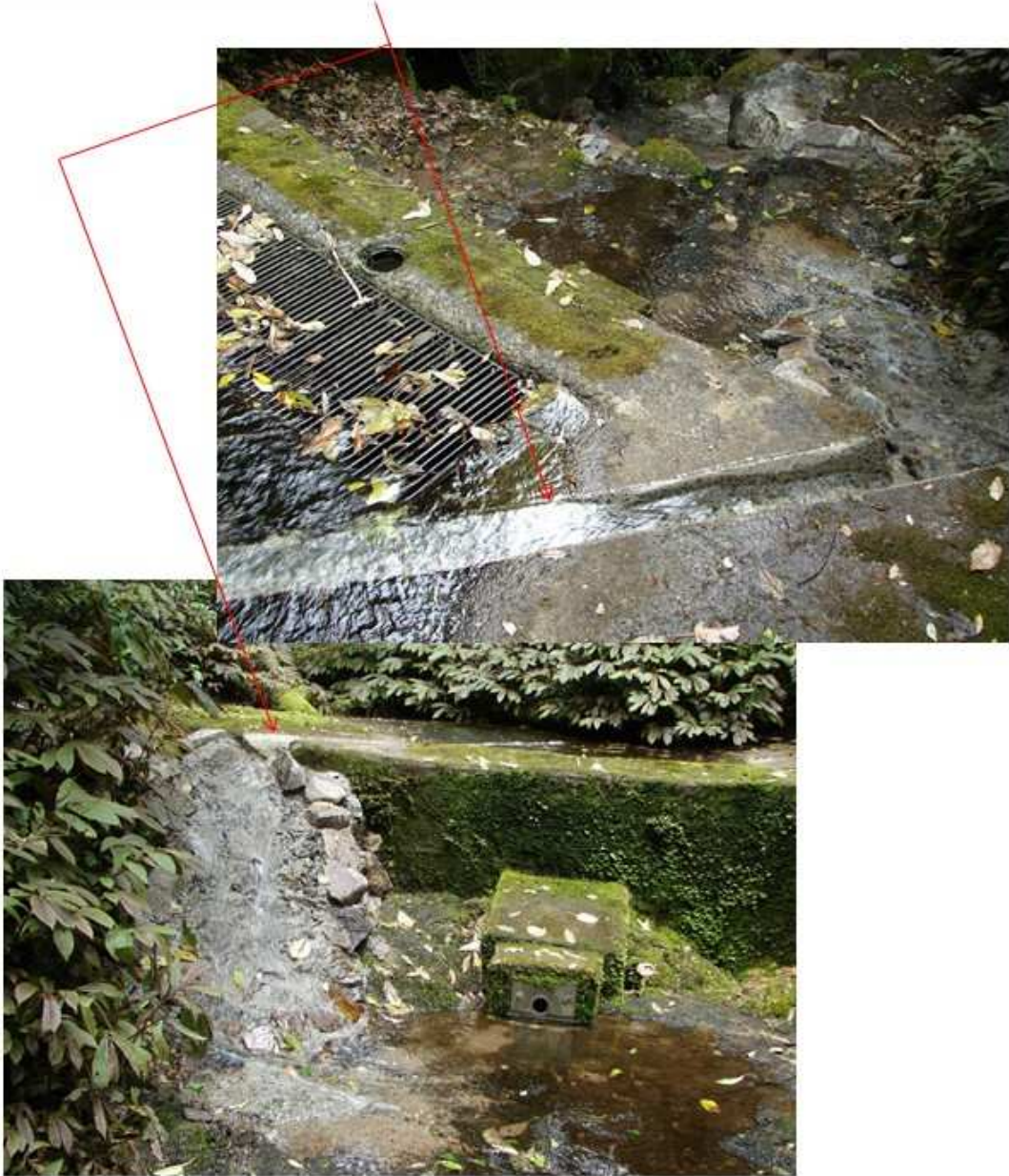
Figure 2-17:Example of a fish pass at Te Aroha. (Text and Photos: Cindy Baker, NIWA)
