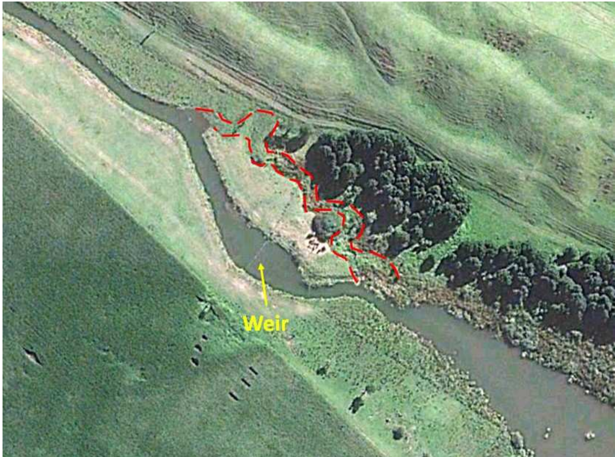
Figure 2-13: Lake outlet and weir. The original stream channel is indicated with broken red lines. [Photo from Google Earth; 9/3/2011].
