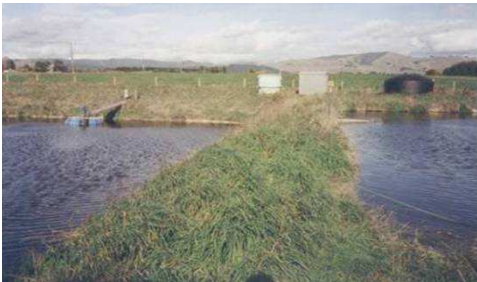
Photo 6. The existing two-pond treatment system of the Massey University No. 4 dairy farm. The anaerobic pond is on the right and the aerobic pond with floating pump is on the left
