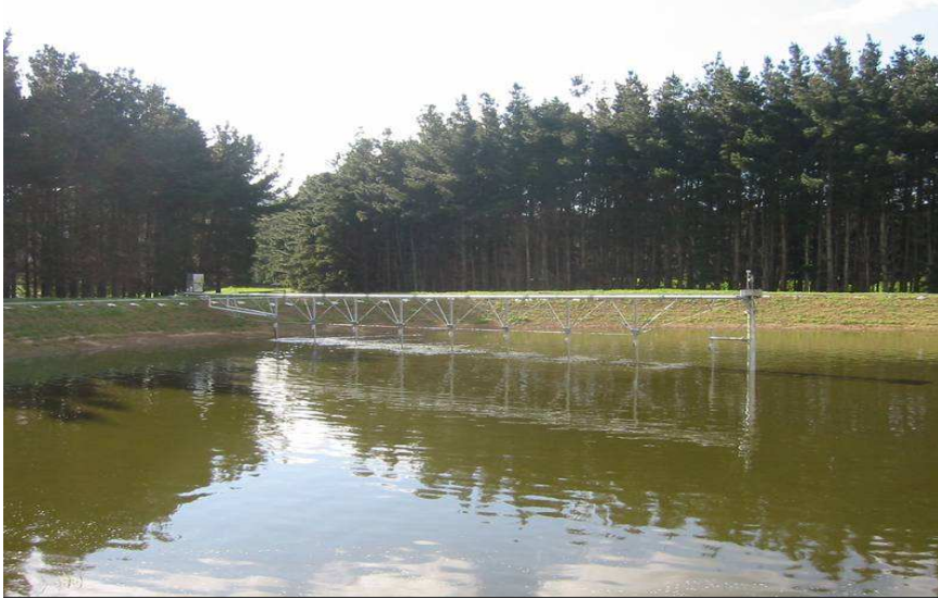
Photo 7. Large effluent storage pond with solids stirrer
