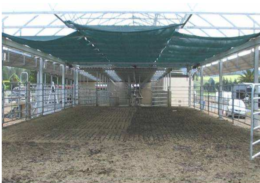
Photo 4. Covered concrete grating of a Herd Home dairy yard.
