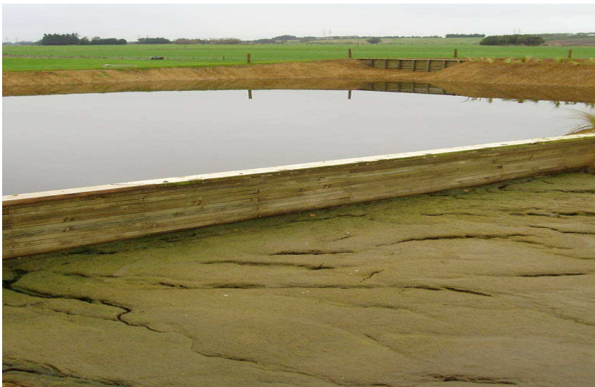
Photo 9. Sludge bed feeding liquid FDE into a large storage pond
