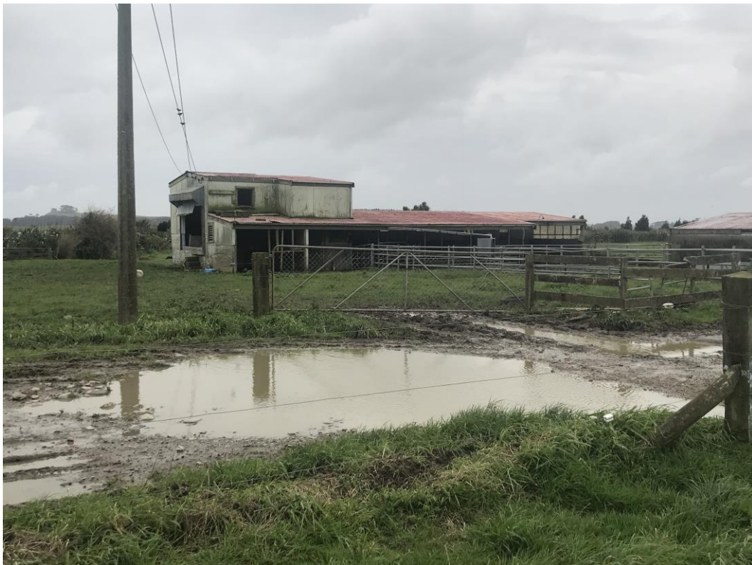
Plate C14: Disused milking shed at 226 Mako Mako Road.
