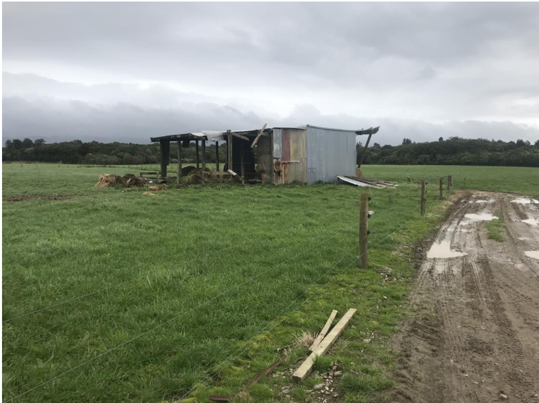
Plate C3: Hayshed at 217 Arawhata Road.
