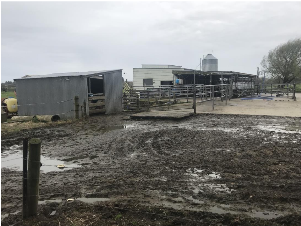
Plate C8: Milking shed at 269 Hōkio Beach Road.
