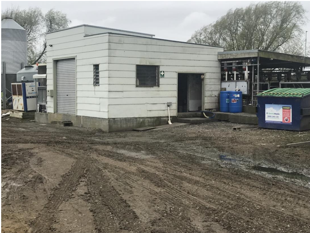
Plate C7: Milking shed at 269 Hōkio Beach Road.
