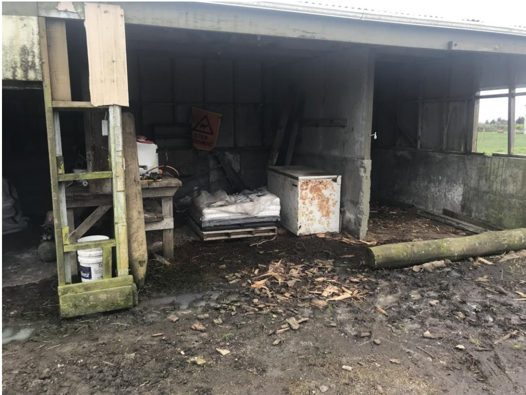
Plate C13: Inside of shed at 215 Mako Mako Road.
