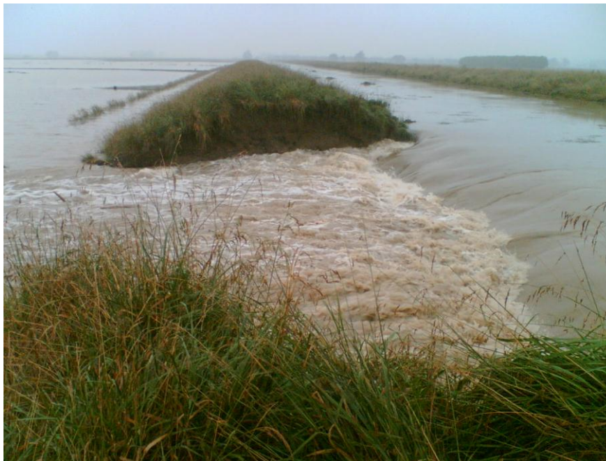
LINTON MAIN DRAIN
