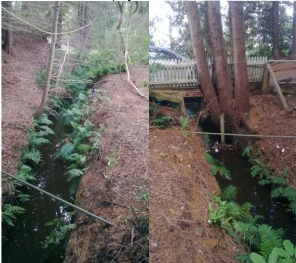
Photos 6.4 & 6.5: Congested sections of Miro Street Drain note severe restriction created by large tree
