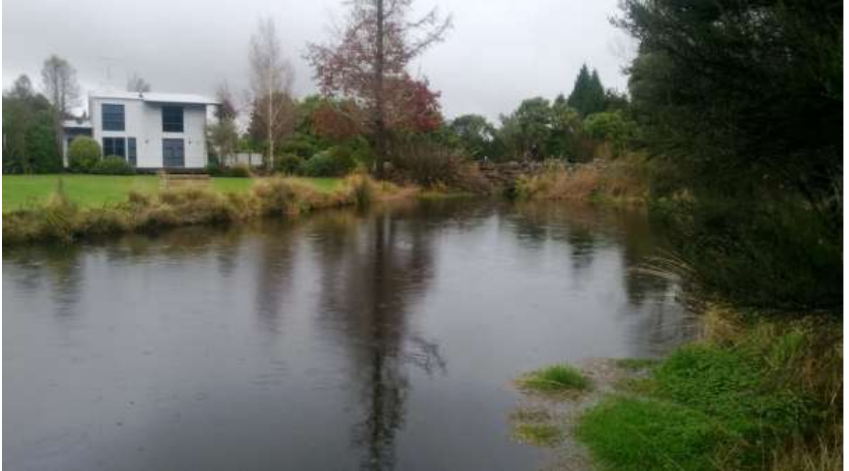
Photo 35: Park Avenue Dam and floodable house
