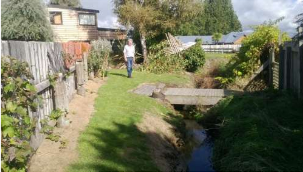
Photo 20: Obstructions to flow and proposed wooden flood wall location adjacent to fence on left bank. Flood wall continues through gap behind green waste to connect into grassed stopbank – in distance.
