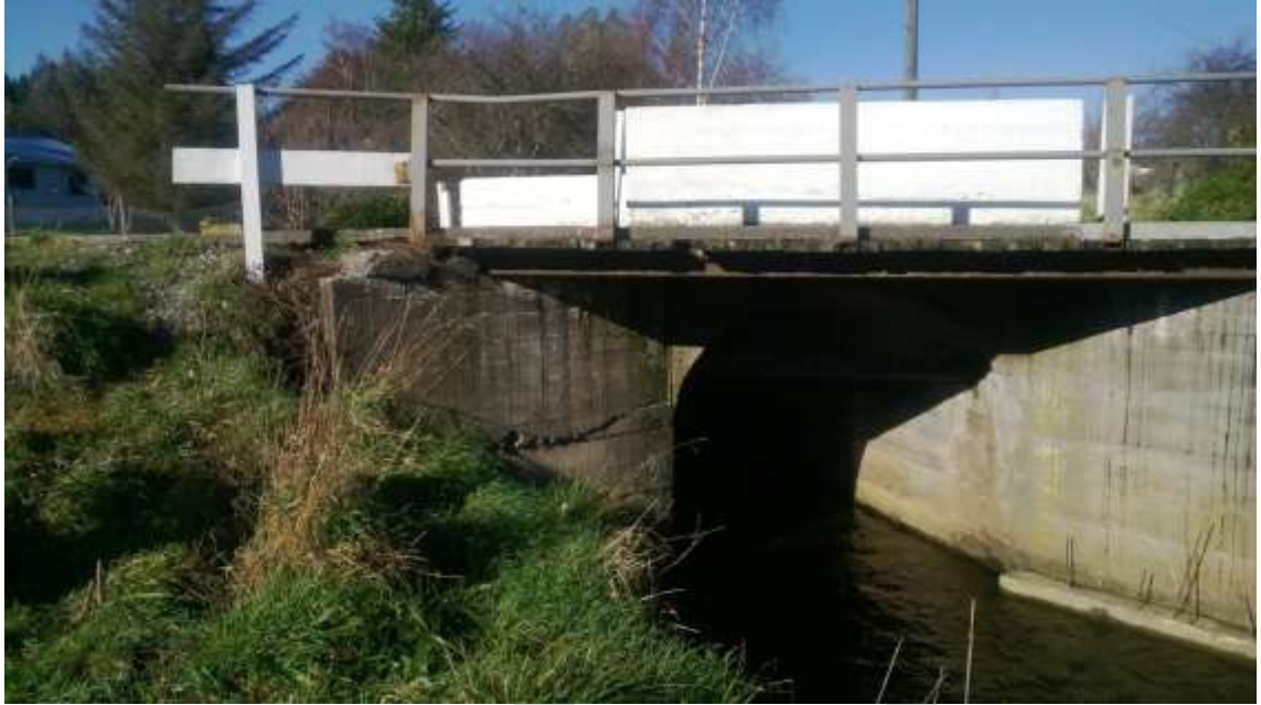
Photo 7.2: Channel A culvert upgrade location at Miro Street
