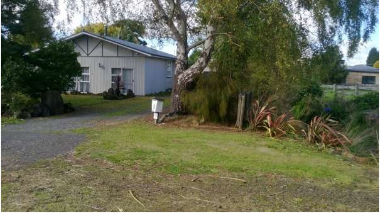
Photo 26: Low-lying house at 2 Martin Place adjacent to Miro Street Drain. A wooden floodwall will have to be constructed through here.
