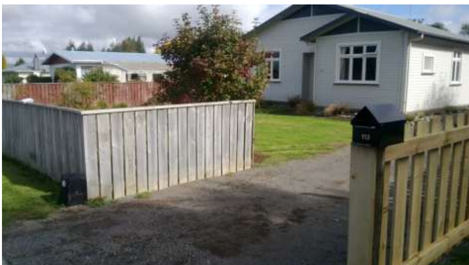
Photo 16: At 113 Miro Street the house floor level is roughly 500mm above the stream bank crest. Freeboard in a 0.5% AEP flood would be small. The culvert crest is around 200mm only below the driveway level.
