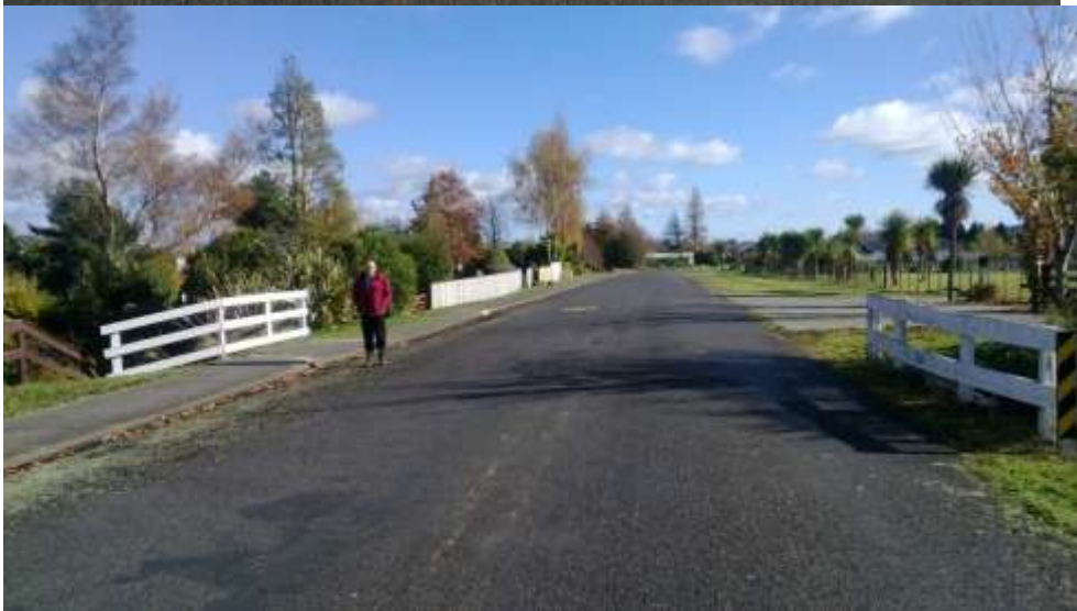
Photos 33 & 34: Shannon Street Culvert crossing showing location of stalled car in 400mm of surging water (Steve Adams standing there) during 15 October 2013 flood.
