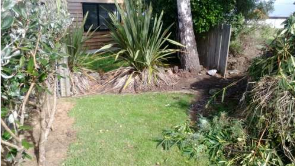
Photo 20: Obstructions to flow and proposed wooden flood wall location adjacent to fence on left bank. Flood wall continues through gap behind green waste to connect into grassed stopbank – in distance.
