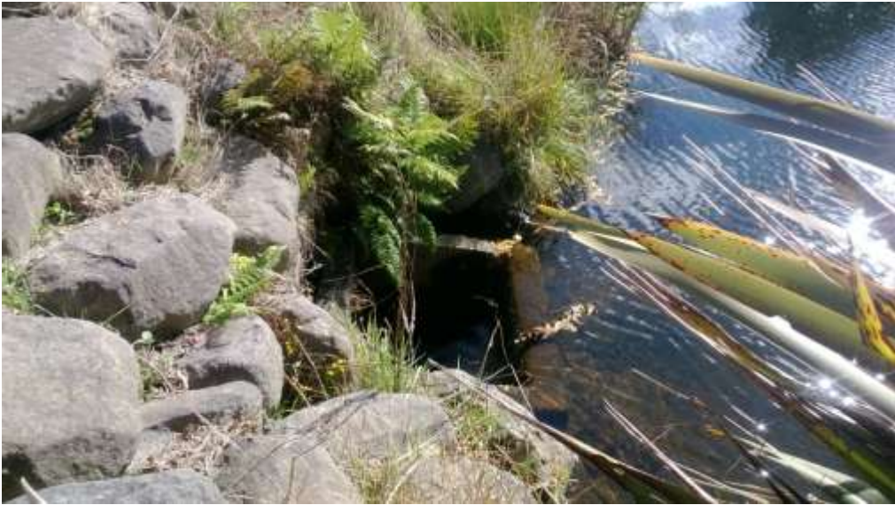
Photo 2: Poor inlet structure to Park Avenue Dam
