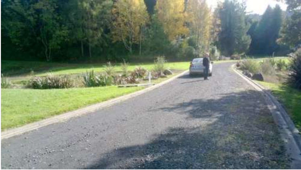
Photos 3 & 4: Dam Crest at Park Avenue
