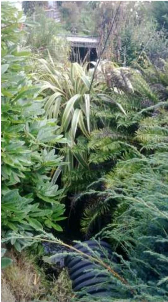
Photo 14: Very congested portion of Miro Street Drain at 115 Miro St, kink in the channel and 450mm diameter corrugated pipe. Photo 15: Channel dimensions at 131 Miro Street.
