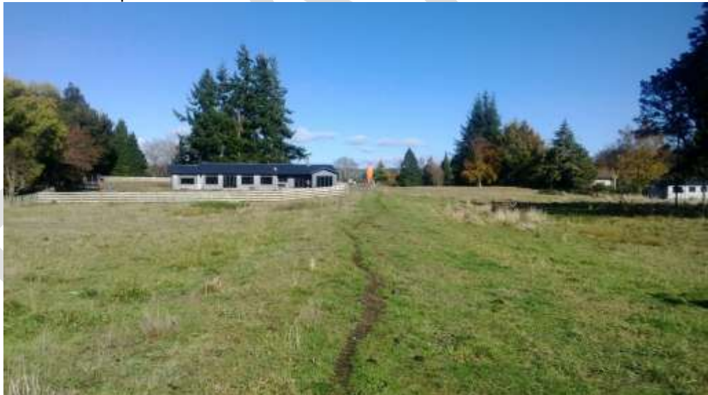
Photo 7.3: Downstream end of proposed Channel B diversion floodway to right of photo
