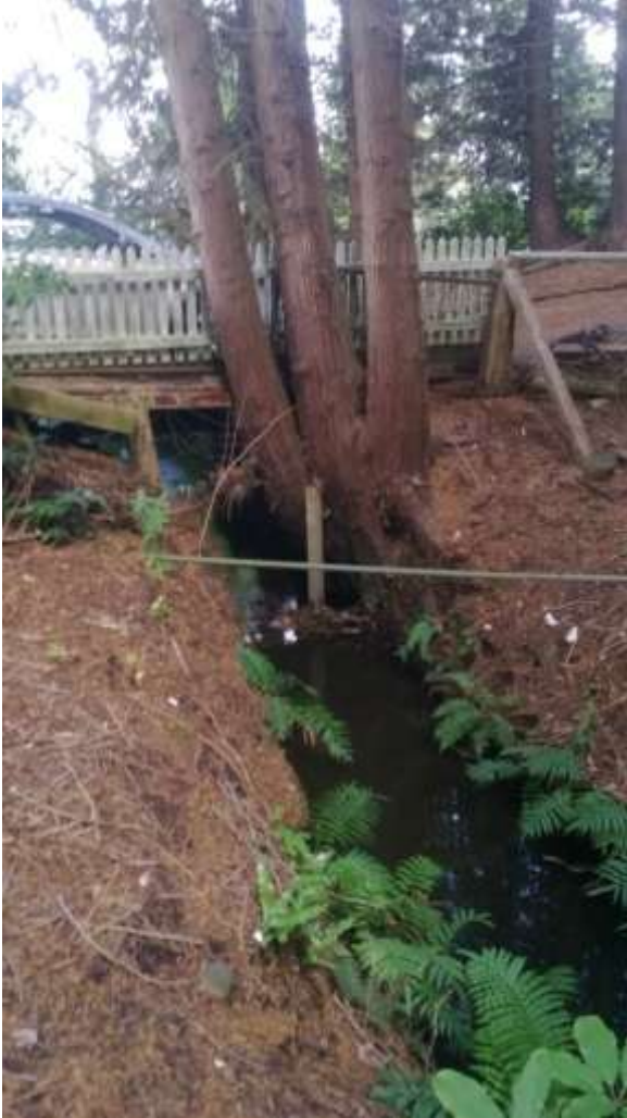
Photo 10: Congested channel at 131 Miro Street, with restrictions due to narrow channel, large trees, low level footbridge and water pipe.
