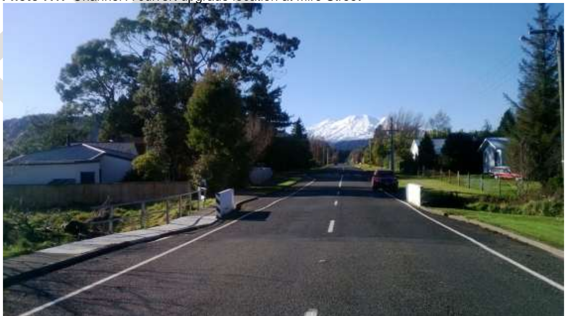
Photo 7.1: Channel A culvert upgrade location at Miro Street
