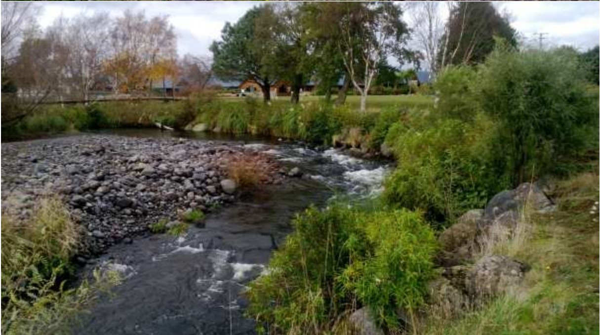
Photos 29 & 30: Sharp bend on Mangawhero River near Mangawhero Terrace & Goldfinch St intersection.
