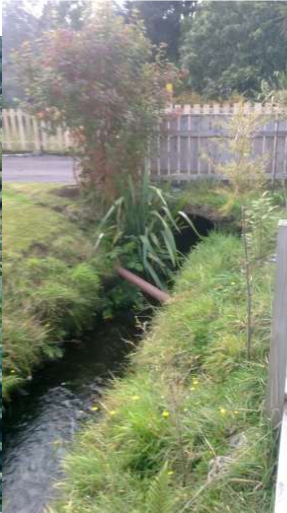
Photo 14: Very congested portion of Miro Street Drain at 115 Miro St, kink in the channel and 450mm diameter corrugated pipe. Photo 15: Channel dimensions at 131 Miro Street.
