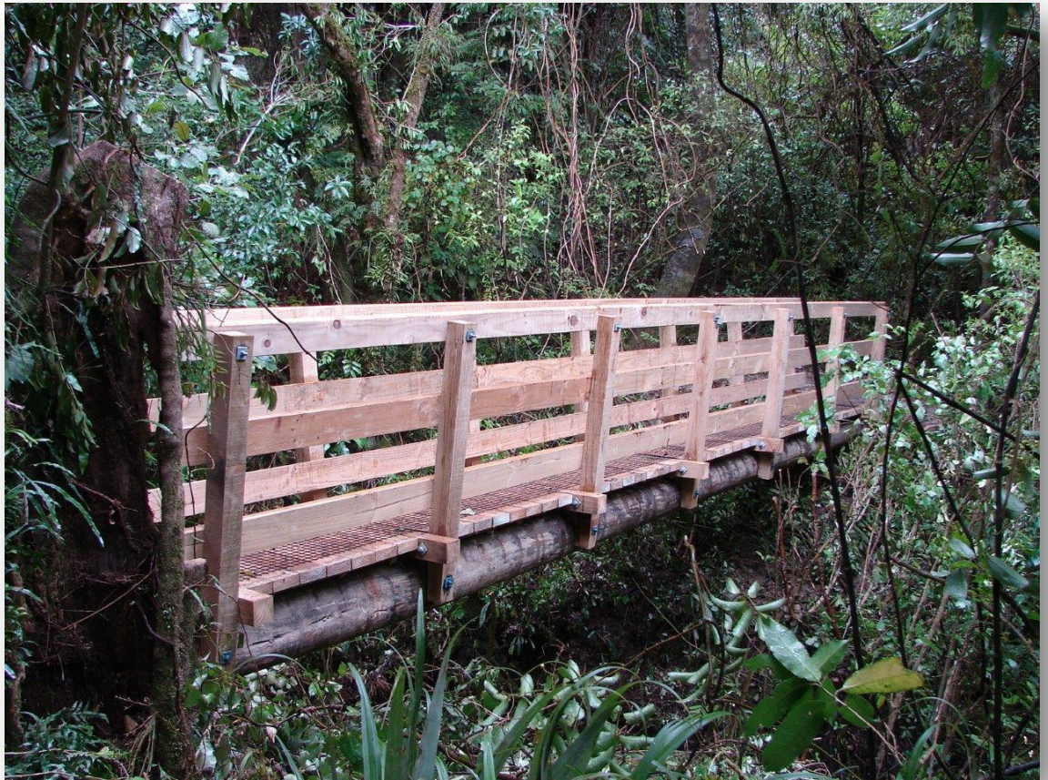
Photo 2: New bridge in the Fern Walk.
