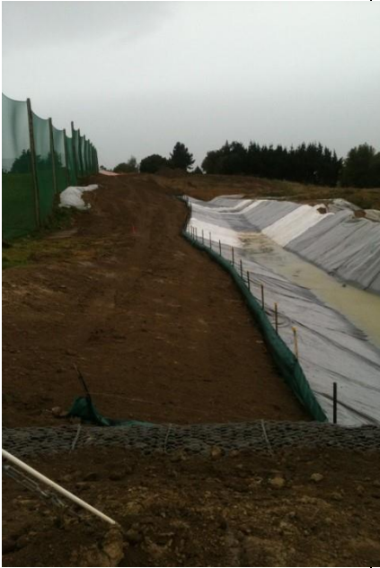
Figure 1. Temporary diversion of water for an earthworks operation
