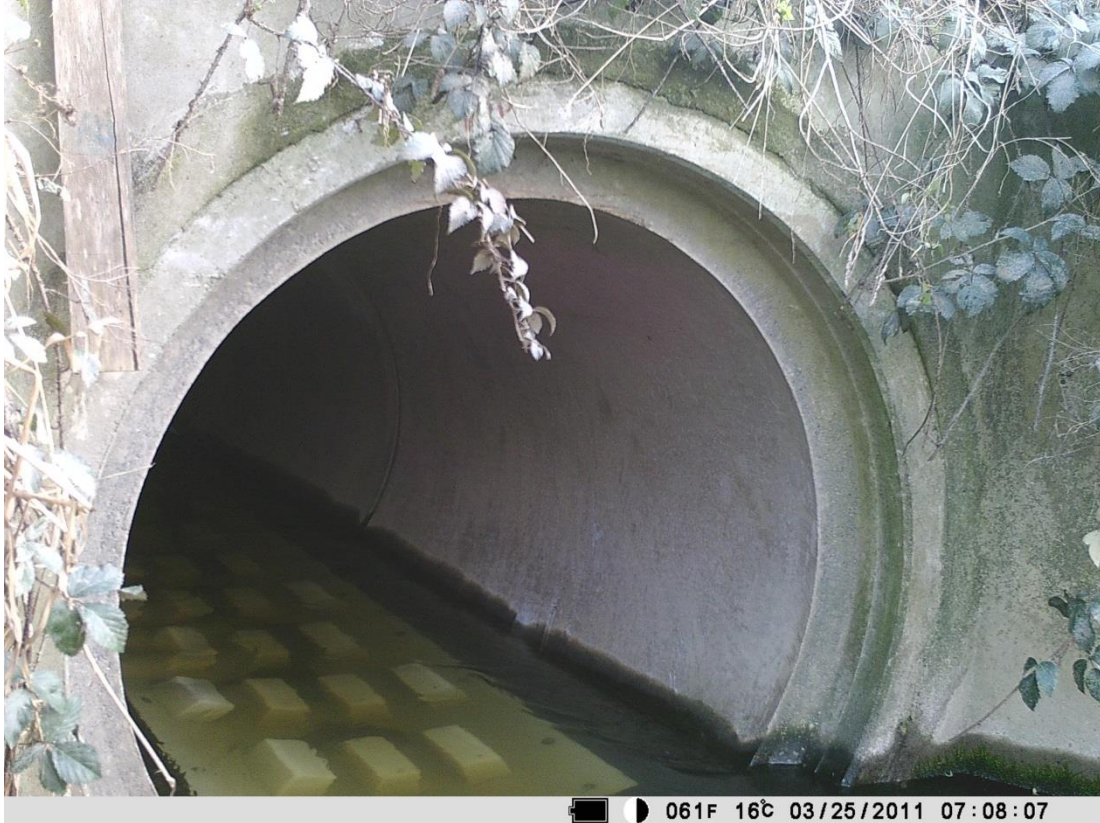
Photo 3 Baffles installed in a culvert on Stantial's drain, a tributary to the Mangaone near Shannon.
