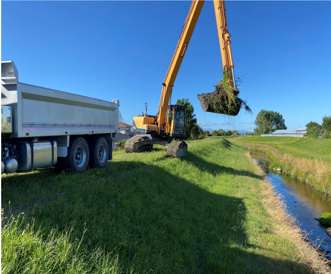
Figure 6: Alligator weed excavation underway at Tremaine Ave Bridge.
