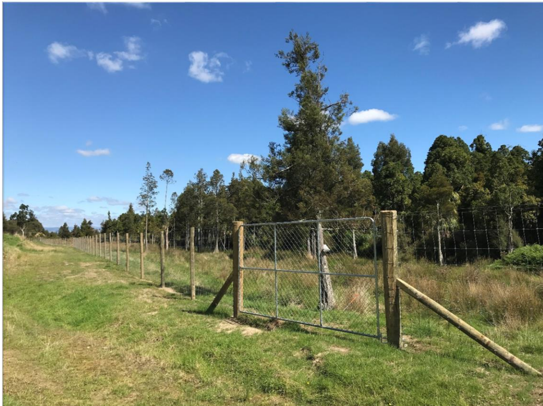
Figure 1: Recently completed deer-proof fence around Broadlands wetland complex. (R.Fleeson)
