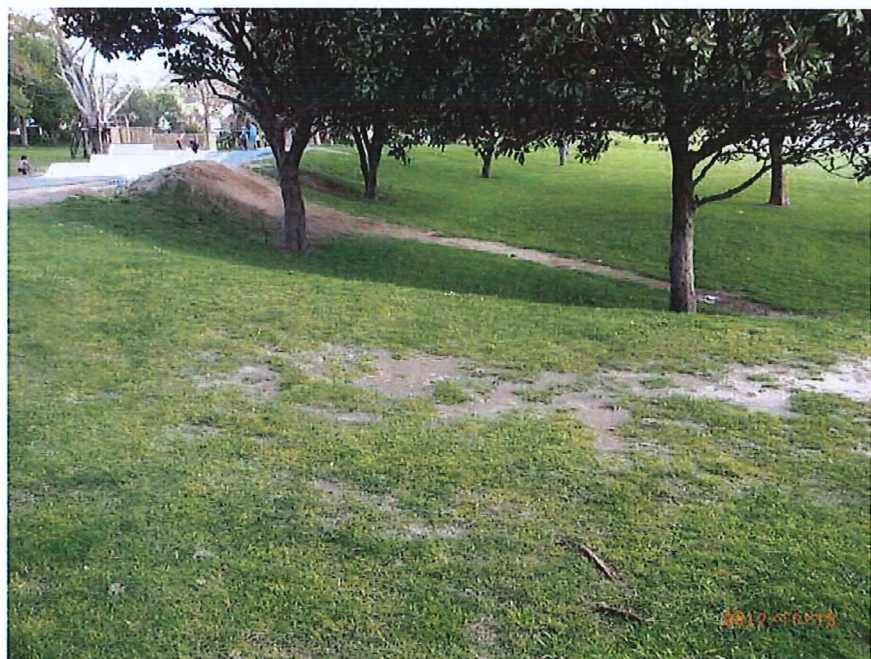
Photo 16: Stopbank damage near skateboard park
