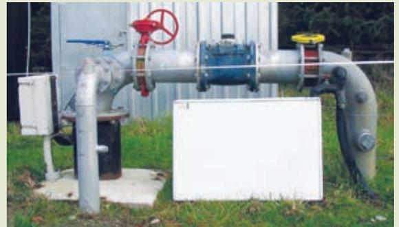
2. Meter too close to flange and gate valve, and insufficient straight length of pipe.
