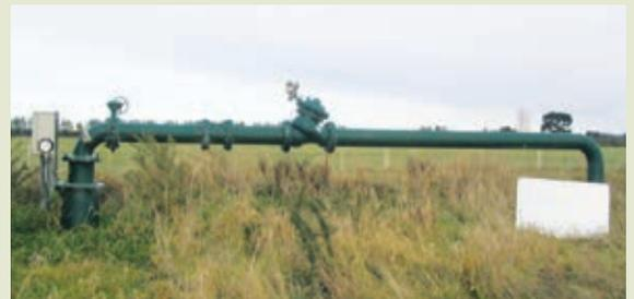
3. Meter too close to control valve and gate valve.
