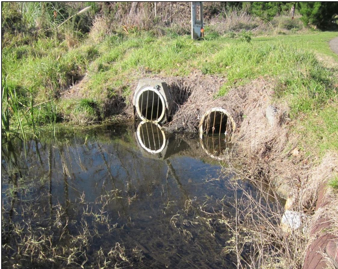
*Figure 1: Photo showing partially submerged outfall and proximity of discharge pipes.*
