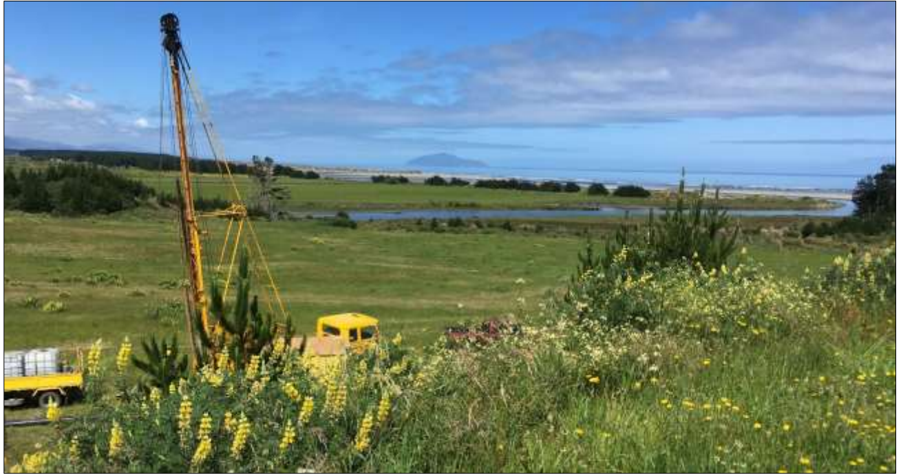
Figure 3. The Neville Webb Welldrilling cable-tool rig drilling the investigation Test Well. View southwest toward the Ohau River, and coastline to the west.
