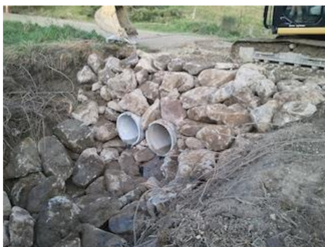
Figure 100 Retaining walls and drainage on a farm track. Retrieved from http://johnstoneng.co.nz/wp-content/uploads/2015/05/Retaining-Walls-and-Drainage.jpg
