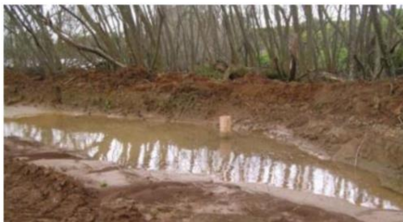
Figure 177 Example of a decanting earth bund. Retrieved from http://www.hortnz.co.nz/assets/Uploads/Auckland-Waikato-ES-Control-Guidelines-1-1.pdf
