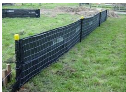
Figure 166 Example of a super silt fence. Retrieved from http://esccanterbury.co.nz/wp-content/uploads/2017/02/sc-super-silt-fence.jpg
