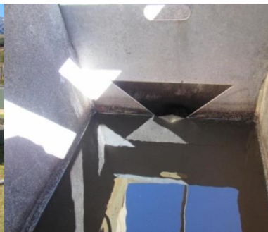
Figure 7 Flow measuring chamber with V-notch weir flow meter
