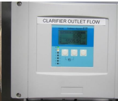
Figure 8 Flow transmitter
