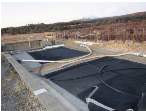
Figure 15 Dewatering pad
