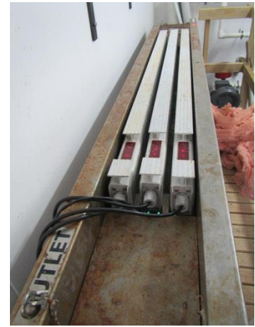
Figure 10 UV disinfection
