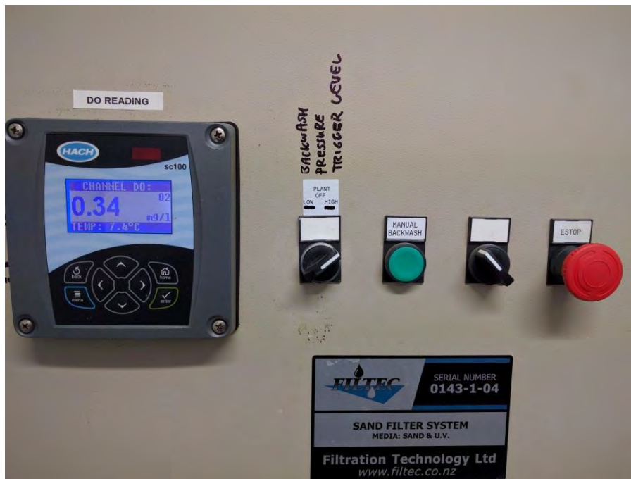
Figure 34 Control Panel for Sand Filters
