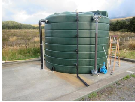
Figure 13 TWAS tank
