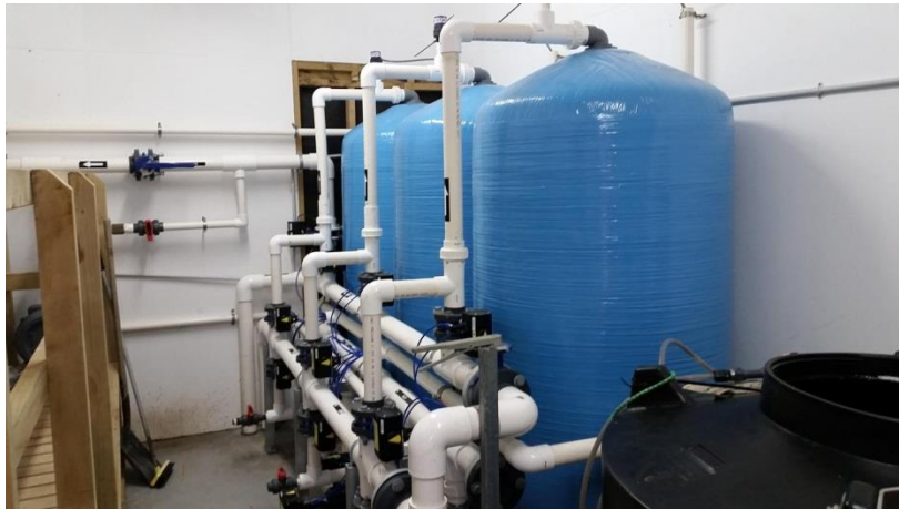
Figure 9 Tertiary filters
