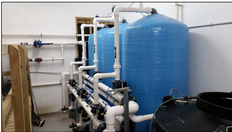
Figure 11 Tertiary filters
