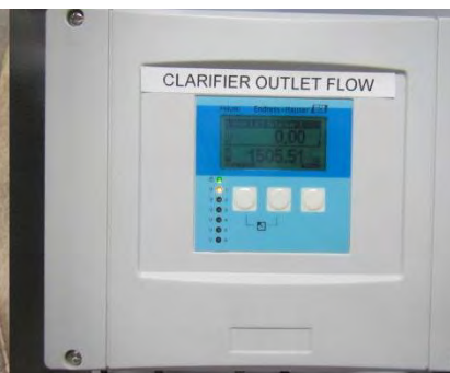
Figure 10 Flow transmitter
