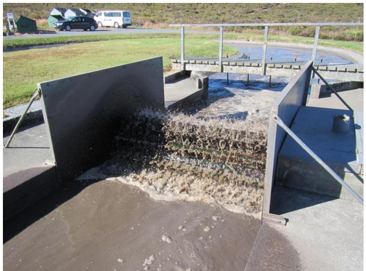
Figure 5 Cage rotor inside Pasveer Ditch
