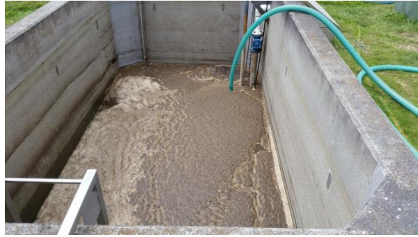
Figure 14 Re-aeration tank
