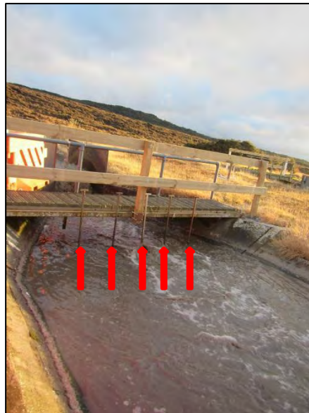
Figure 24 Pasveer Channel with Rag rakes
