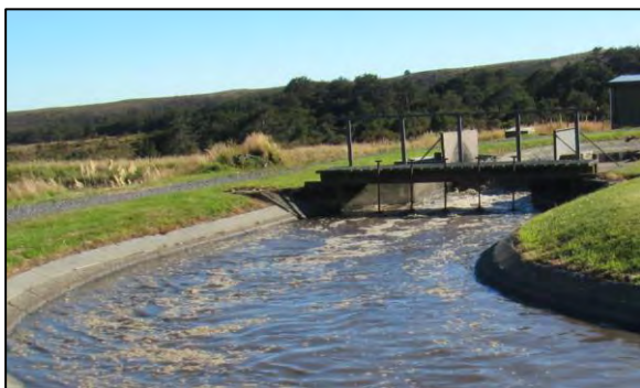
Figure 19 Foam indicating good condition
