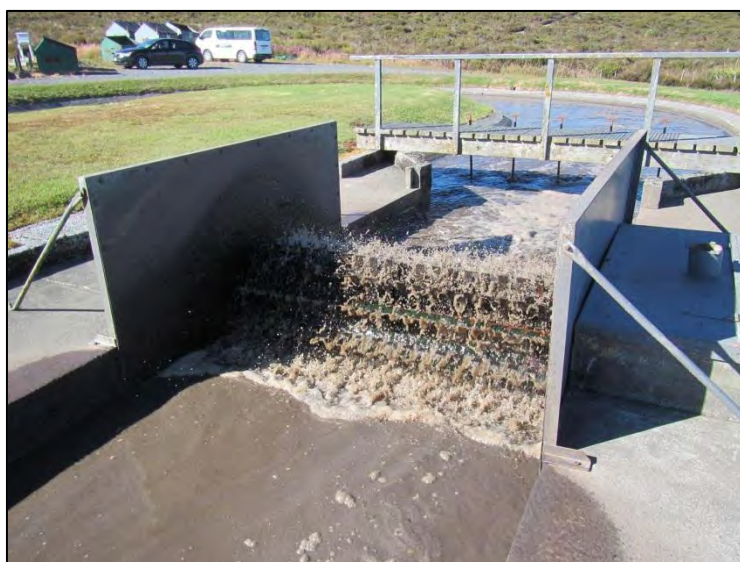
Figure 7 Cage rotor inside Pasveer Channel
