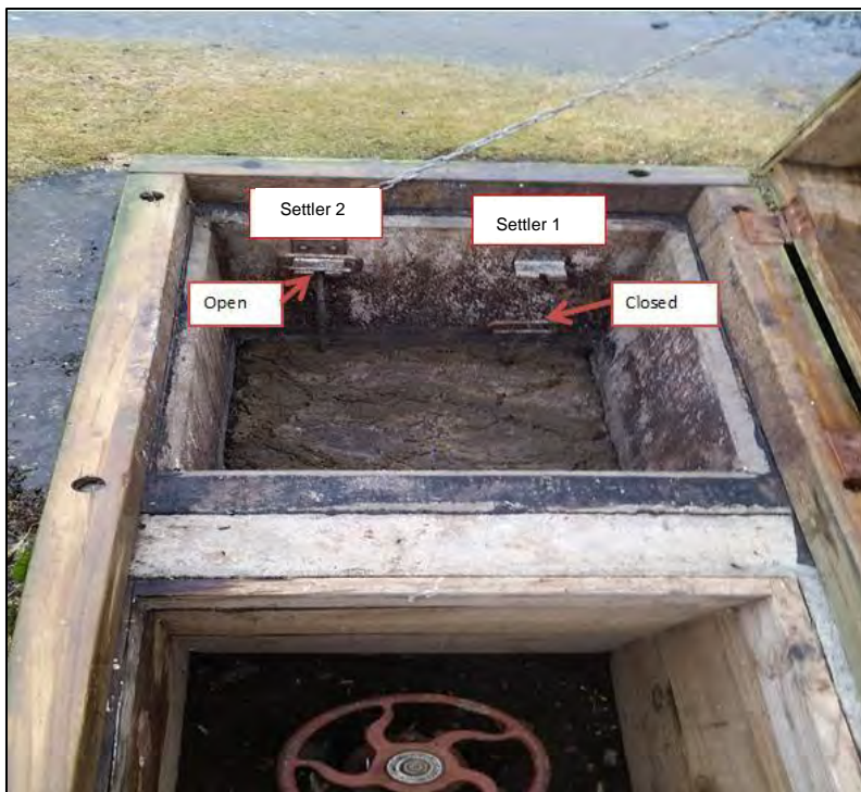
Figure 32 Flow splitter with Valves to control inflow to Settlers
