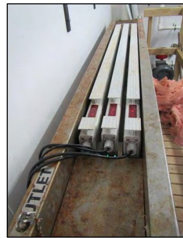
Figure 12 UV disinfection
