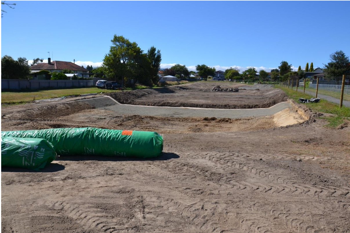
Figure 3 Norton Park wetland under construction with GCL installed beneath topsoil
