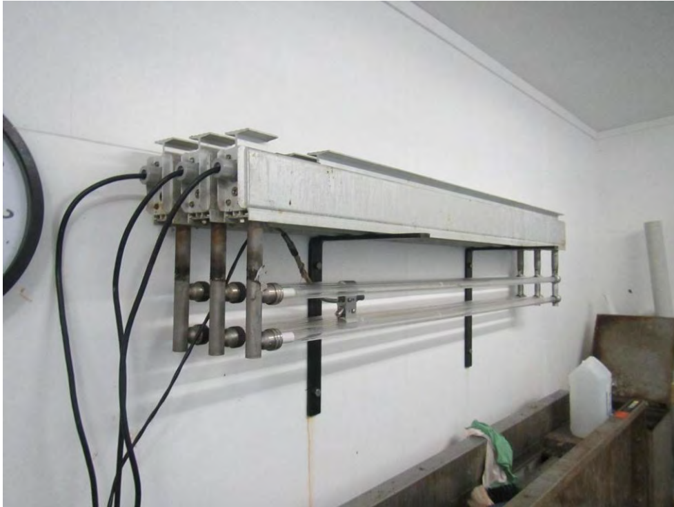
Figure 25 UV system ready for maintenance
