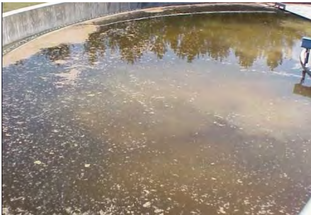
Figure 33 Example of Floc on top of a settler (photo not from Whakapapa)
