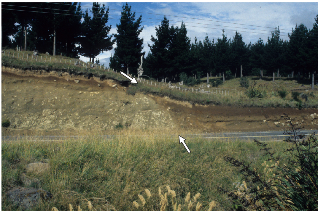
Figure 5.3 Exposure of the active Snowgrass Fault in a State Highway 1 roadcut near Iirangi, identified by white arrows. The fault forms the sharp break between light grey Tertiary rocks and orange-brown Late Quaternary lahars and tephra deposits, mostly from Mt Ruapehu. The scarp, highlighted by the fenceline, is c. 5 m high. Photo credit: Pilar Villamor.
