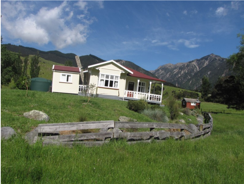
Figure 1.2 A house built along the scarp of the Papatea Fault in the Clarence River valley, Kaikōura District. The scarp is broadly defined by the pre-existing fence and line of boulders. Surface rupture across the fault in the 2016 Kaikōura earthquake resulted in vertical and horizontal ground deformation that warped and tilted the ground (to the right), damaging the house and causing the chimney to separate from it. There were no occupants in the house at the time of the earthquake. Image from Van Dissen et al. (2019).
