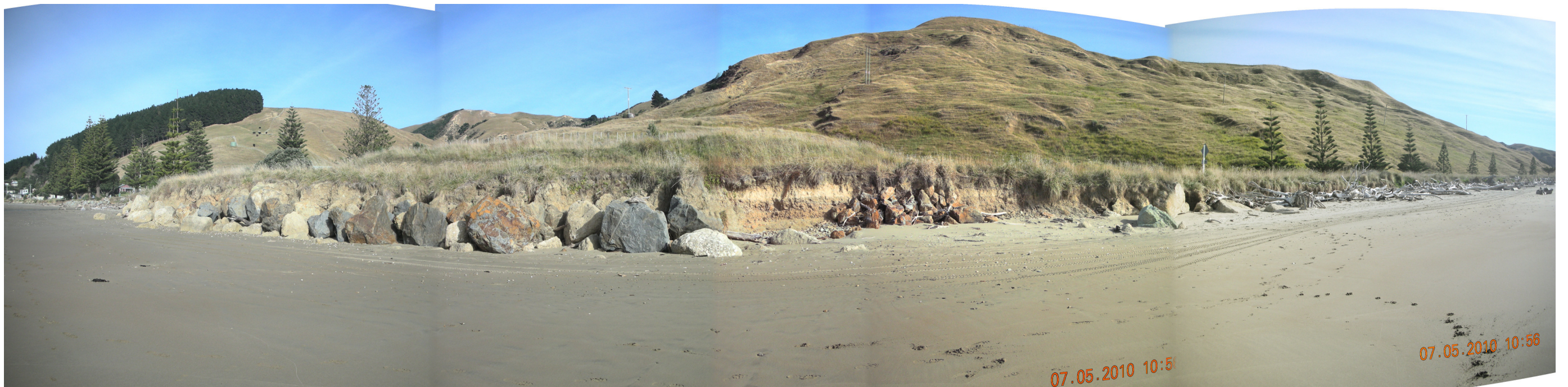
Photo 5 looking west showing protruding shoreline with placed rock protection and recent erosion scarp exposing slip debris backshore.
