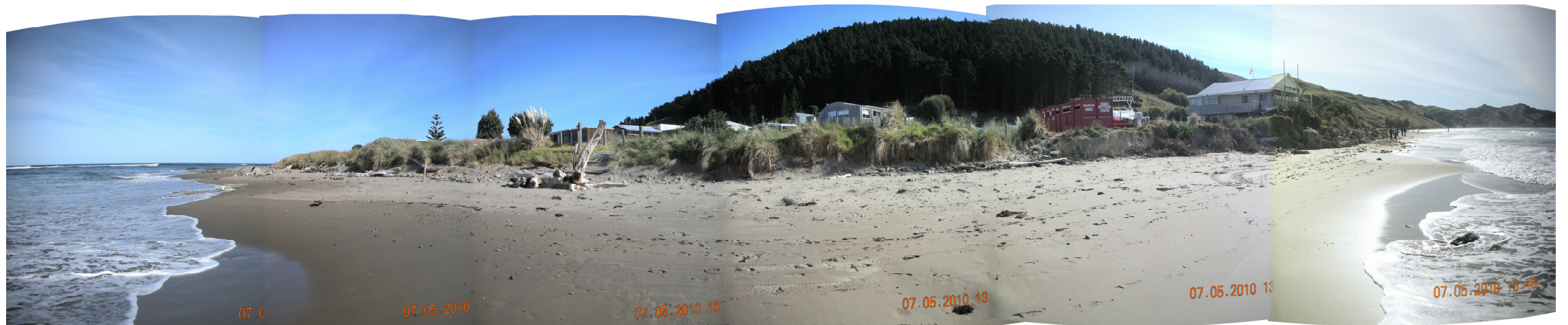
Photo 8 looking west showing area in front of the camp ground. Note localised erosion (end effects) at end of the rock protection.
