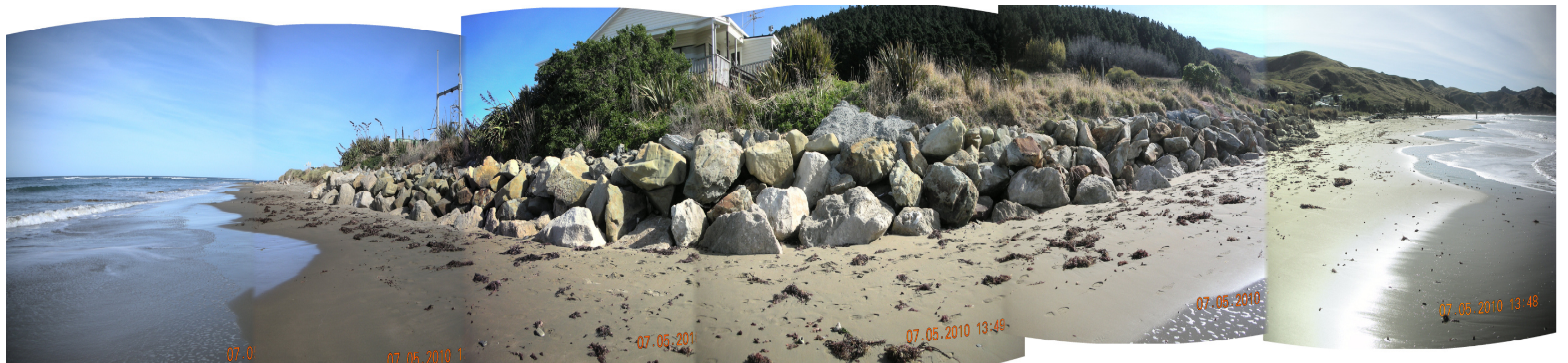
Photo 9 looking west showing rock erosion protection in front of the boat club.
