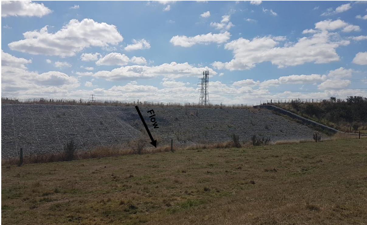
Figure 3: Photograph of Gabion Drop Structure (20 March 2019)
