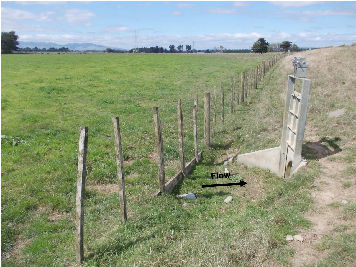
Figure 8: Photograph of Circular Conduit Provided across Stopbank taken from Upstream Right Side (20 March 2019)
