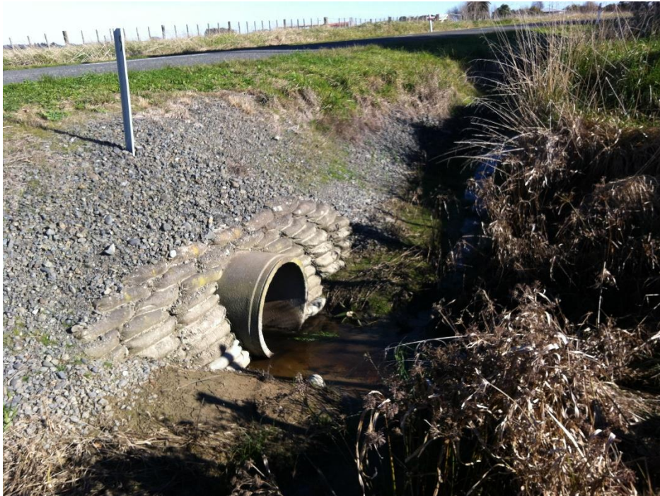
Figure 1 Typical table-drain culvert, Rowe Road
