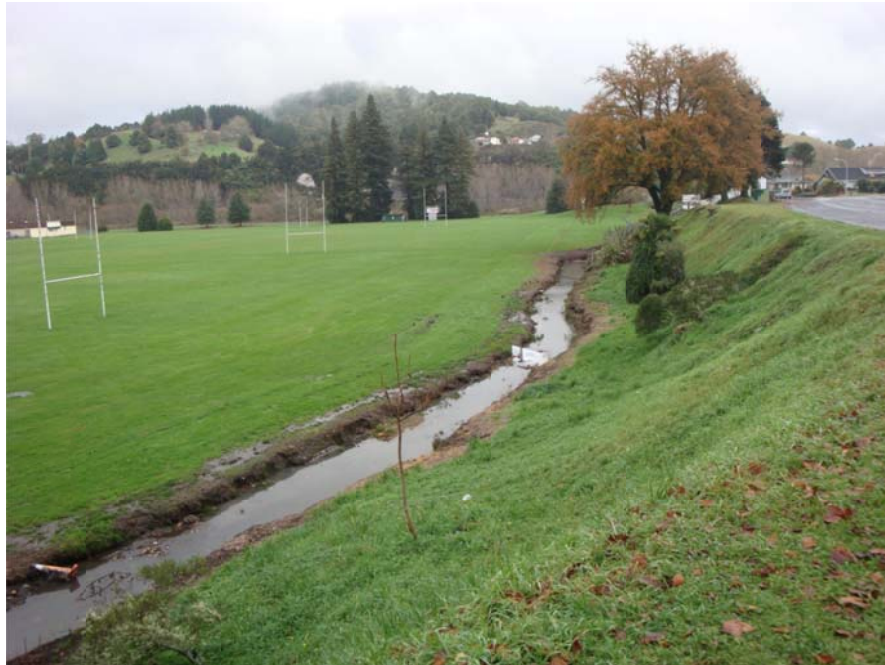
Figure 5-4: Open drain with no stopbanks: Taumarunui Domain, adjacent to Morere Terrace
