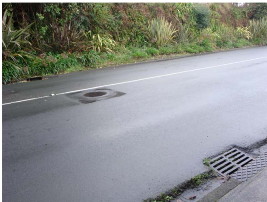
Figure 5-6: Typical catchpit found in Taumarunui stormwater network
