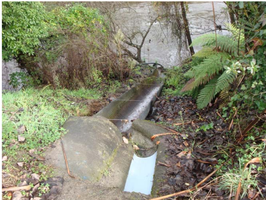
Figure 5-5: Stormwater pipe discharging into the Ongarue River
