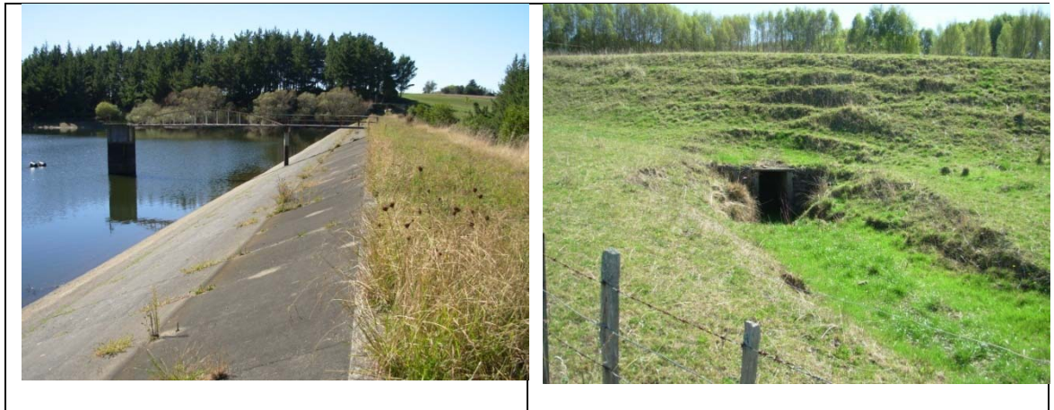
Figure 4-4 Water supply dam wall (left) and dam W8 outlet (right)
