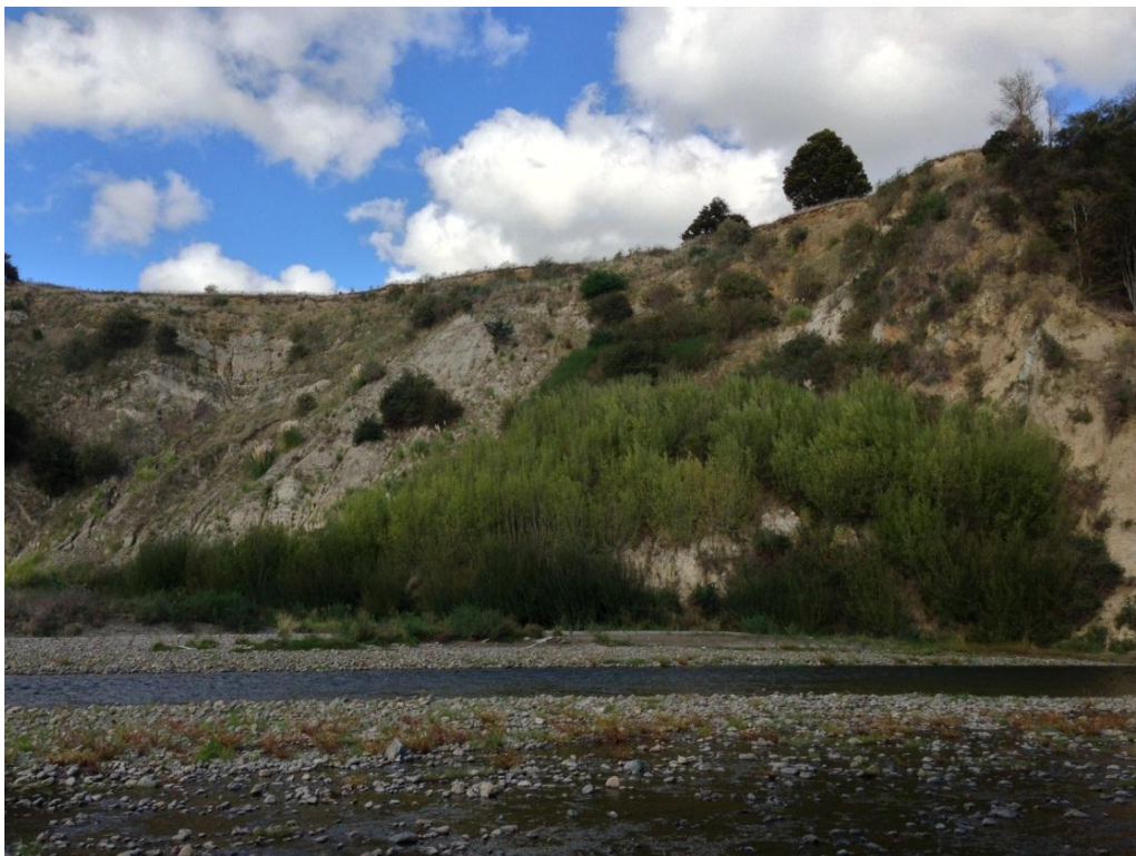
Photograph 8: Currently stable slip on left bank at river distance 17.2-17.3 km
