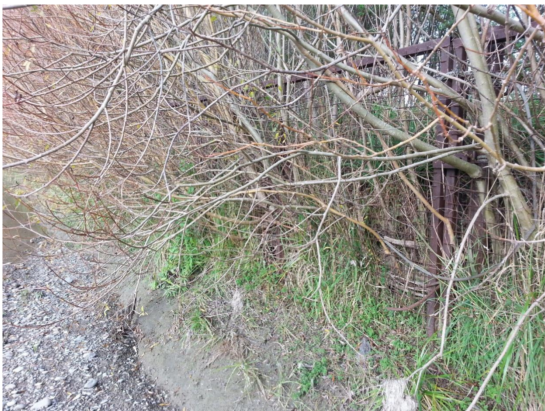
Photographs 13 & 14: PMUs providing good riverbank protection on left bank river distance 9.5 to 9.8 km
