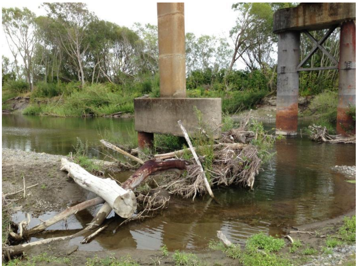
Figure 15: Rail Bridge abutments
