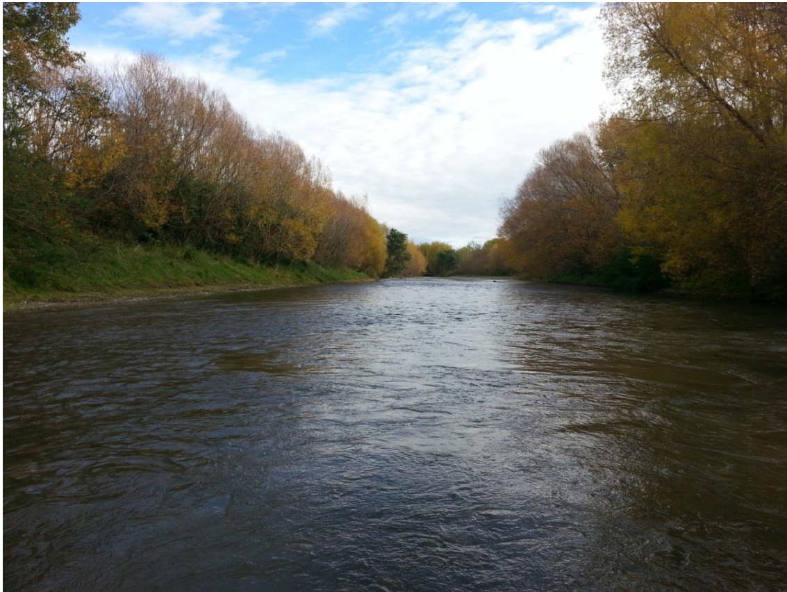
Photograph 12: Scheme in very good condition looking downstream from Almadale Road at river distance 12 km
