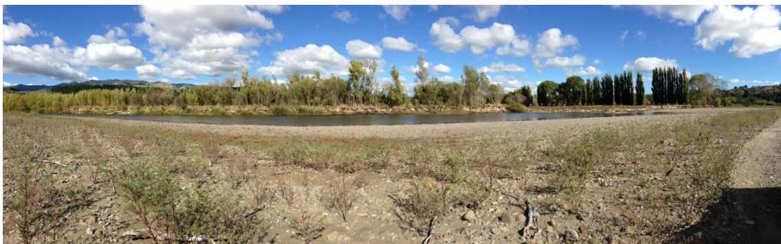
Photograph 5: Panorama of erosion on left bank at McDonald river distance 14.2-14.8 km
