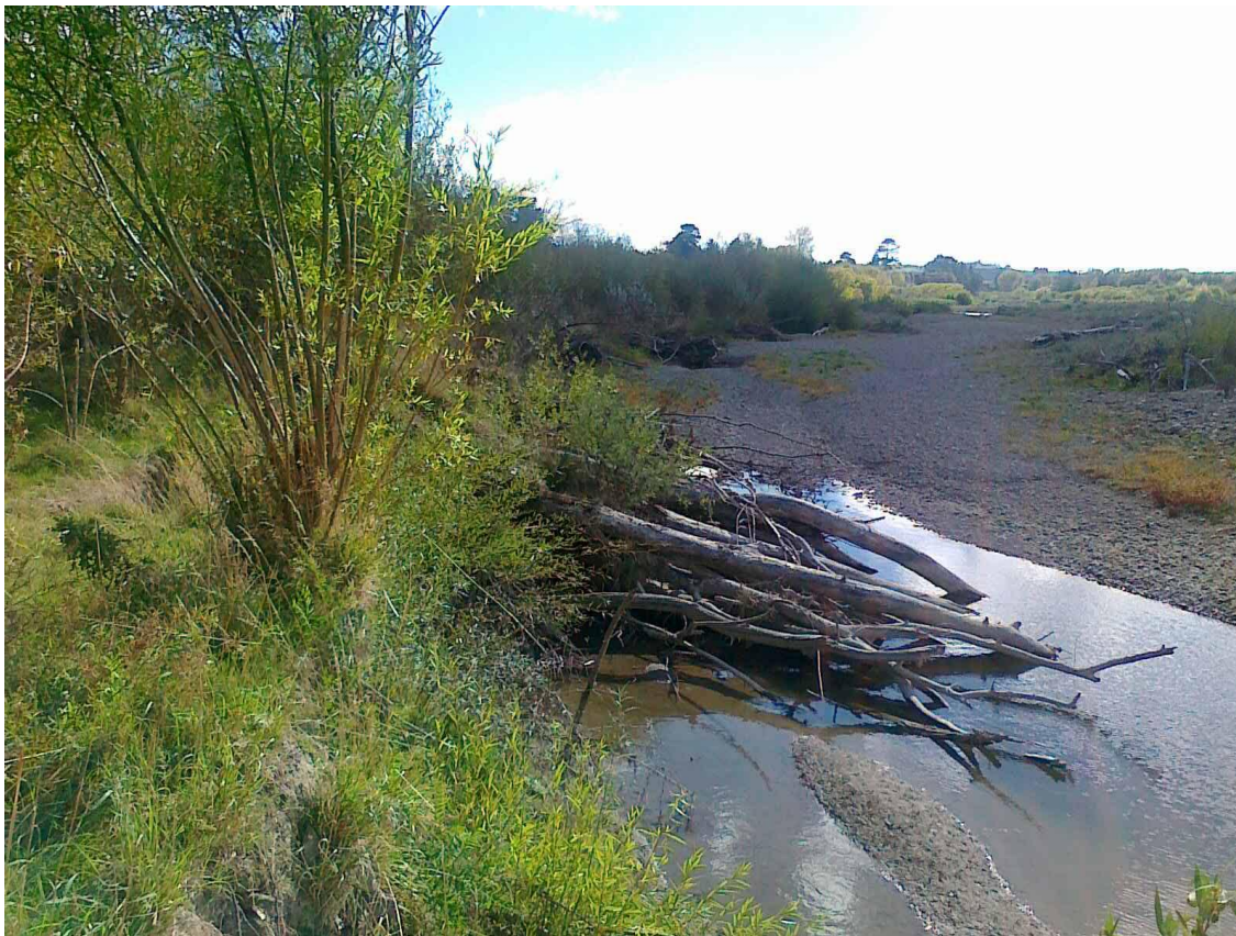
Photograph 3: Established tree groyne on right bank at 7.2 km.
