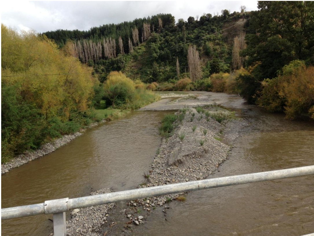
Photograph 1: Looking downstream from Londons Ford Bridge. MDC water intake on left bank in channel that is periodically cleared and gravel redistributed. River distance 40.7 km.
