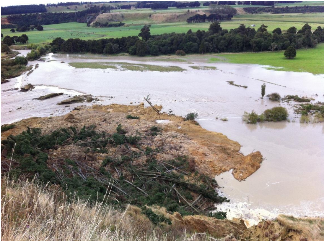
Photograph 7: Large slip off forestry block at river distance 20 km
