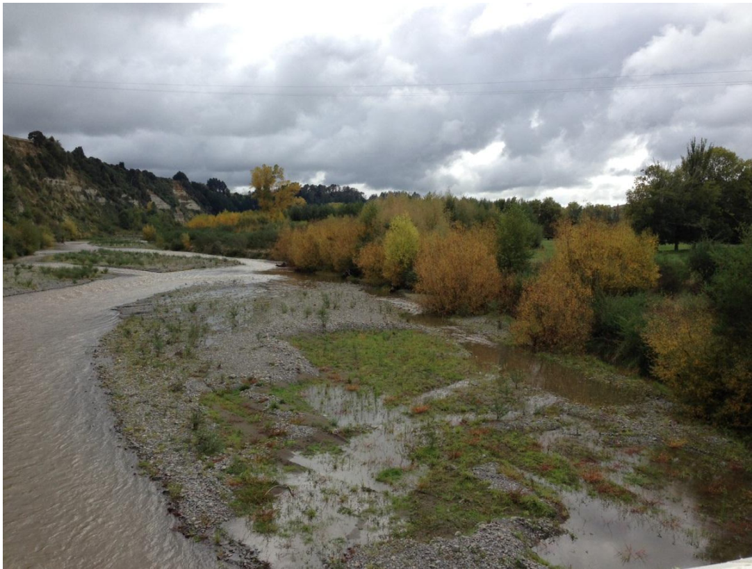
Photograph 2: Aggraded beaches 39-40 km reach. Need to be kept clear of vegetation and lowered.
