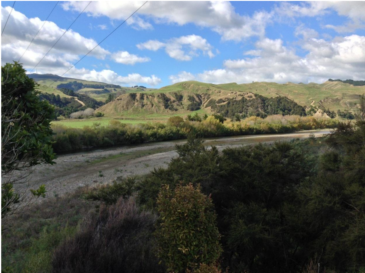
Photograph 1: Stable left bank opposite with Akers groynes from pylon 4 to 4.8 km
