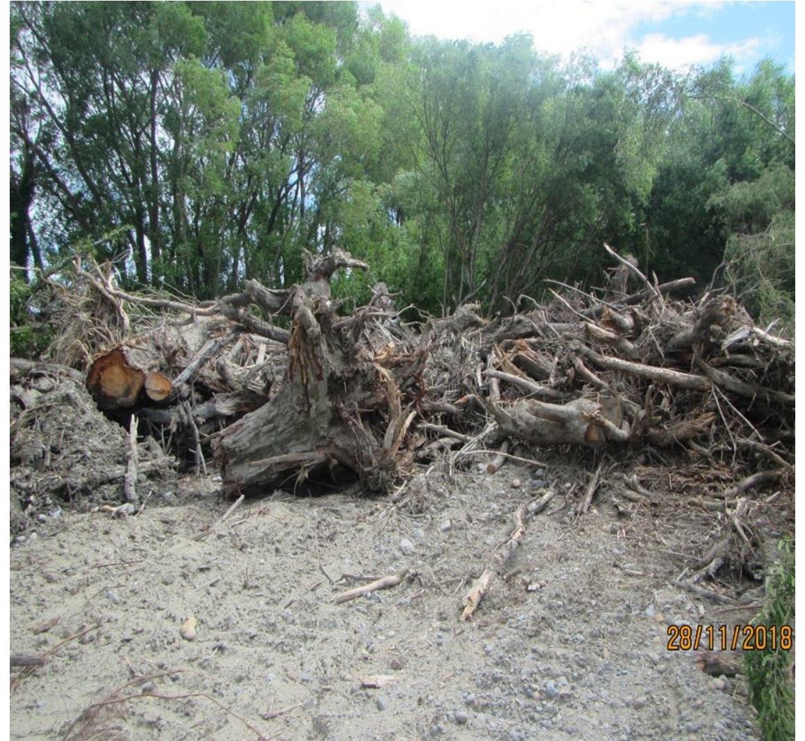
Clearing the large volumes of debris removed from the active channel
