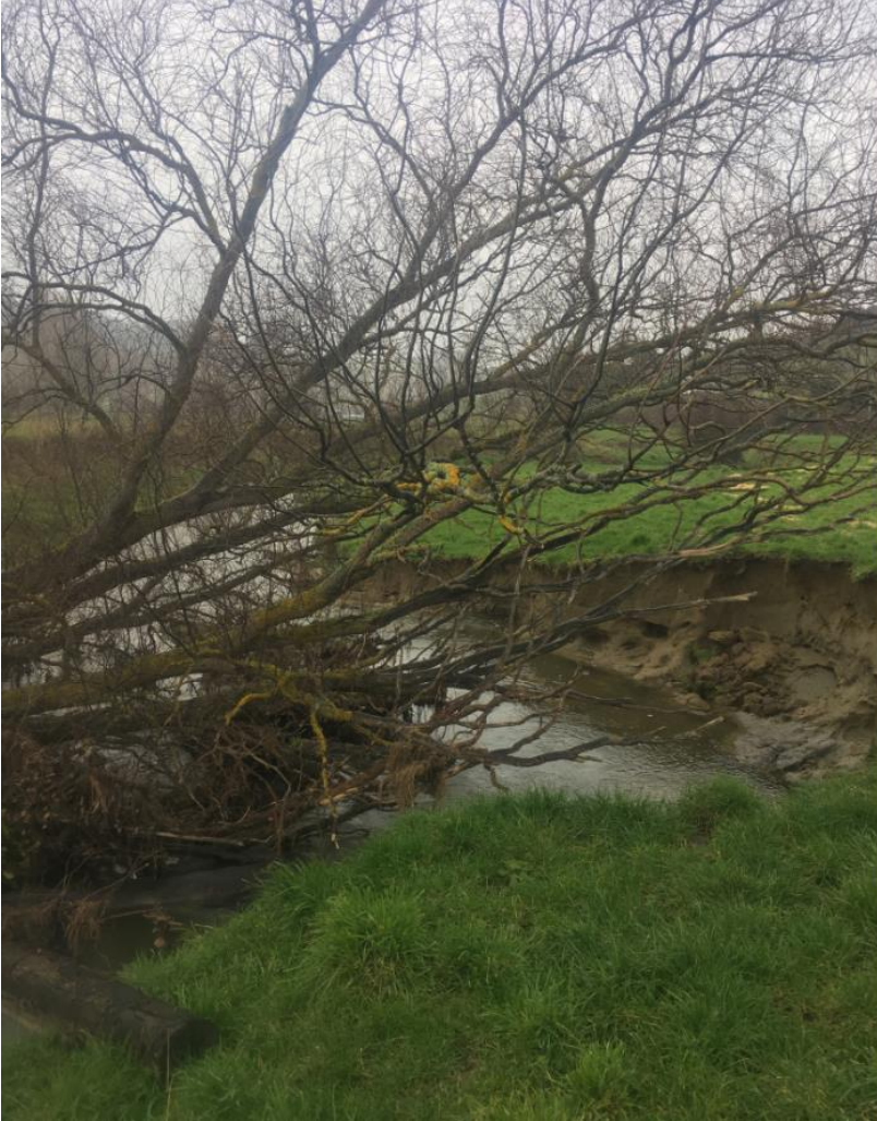
Tree blockage just south of Hunterville (since removed)
