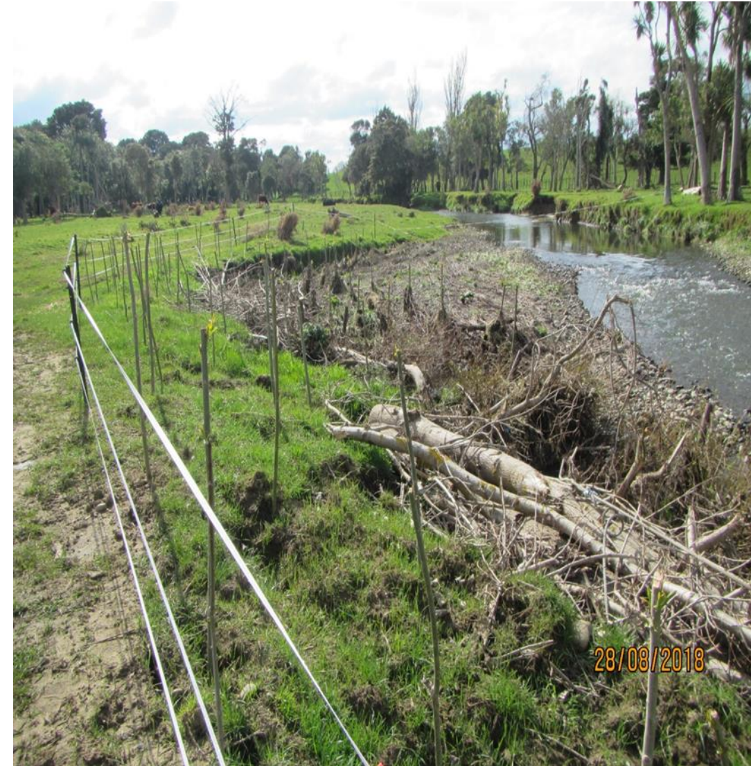
Typical willow planting at a repair site
