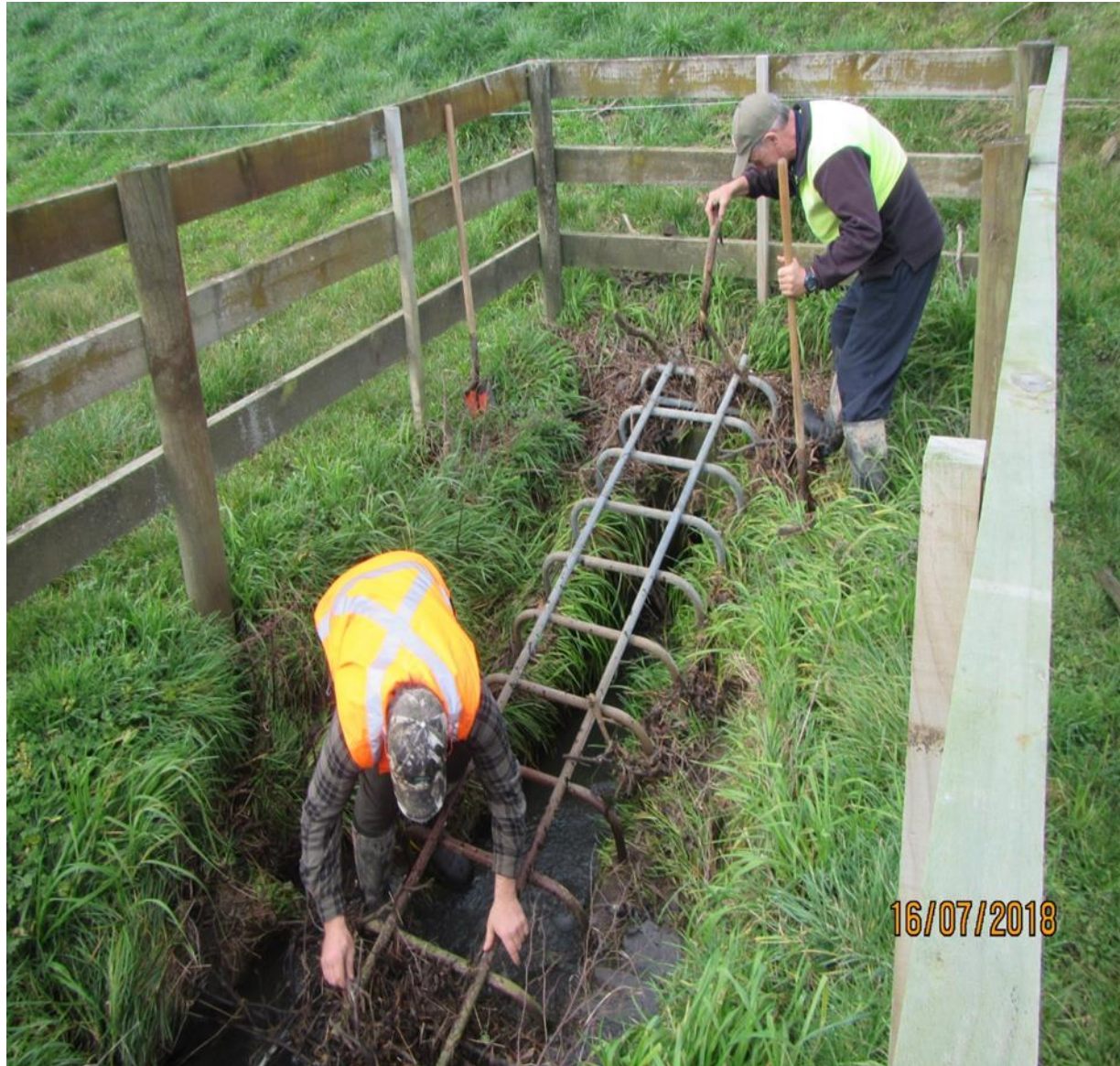
Typical grate clearing operation by our staff
