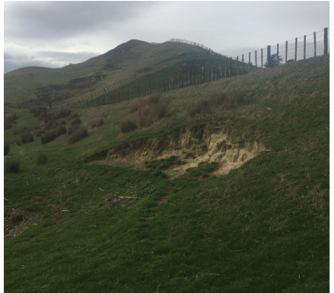
An example of stock tracking on the dam embankment. We plan to address these issues when it can be fitted into the budget
