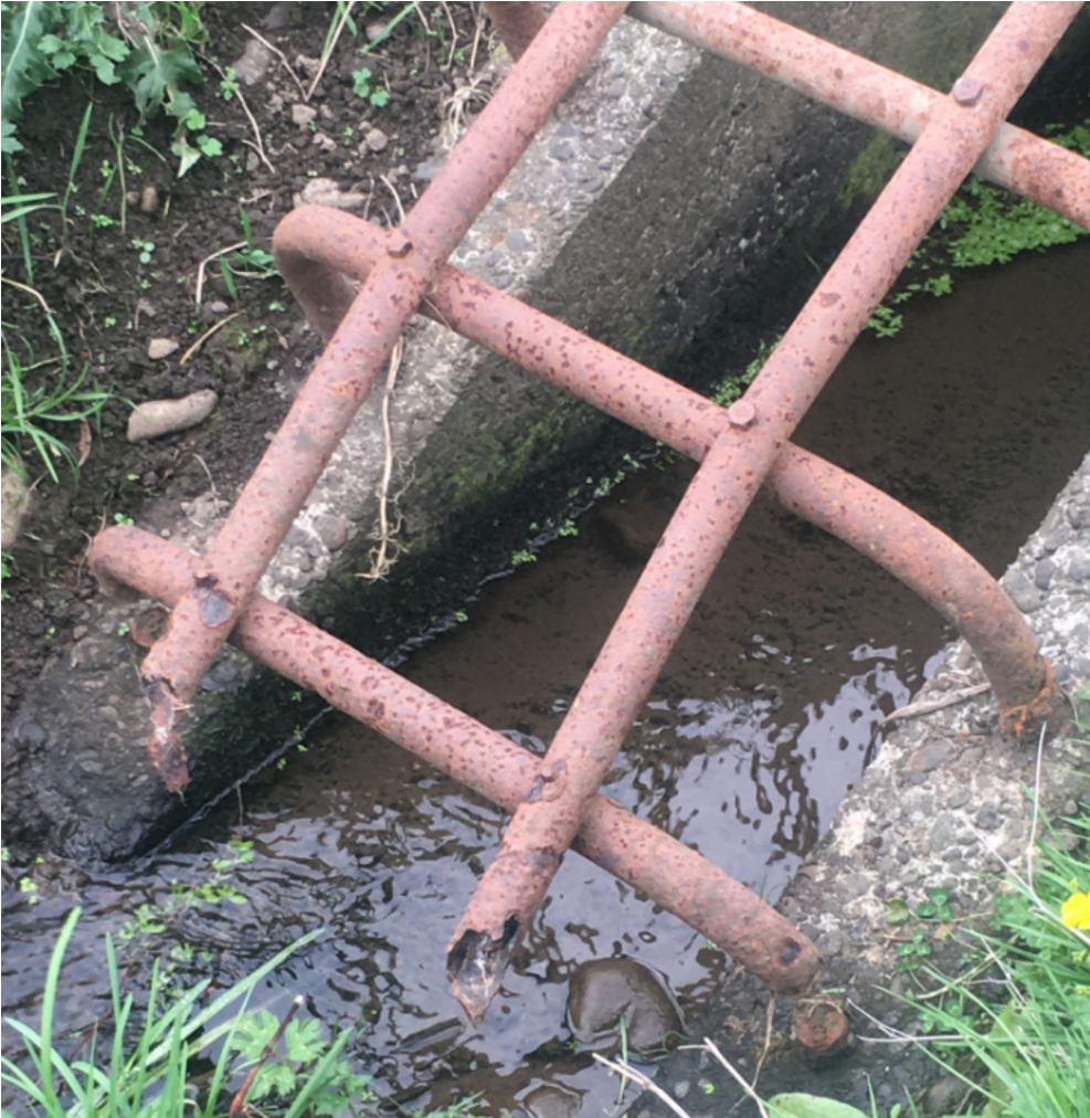
Dam 39, an example of a number of inlet screens which are rusted and due for replacement in the next few years
