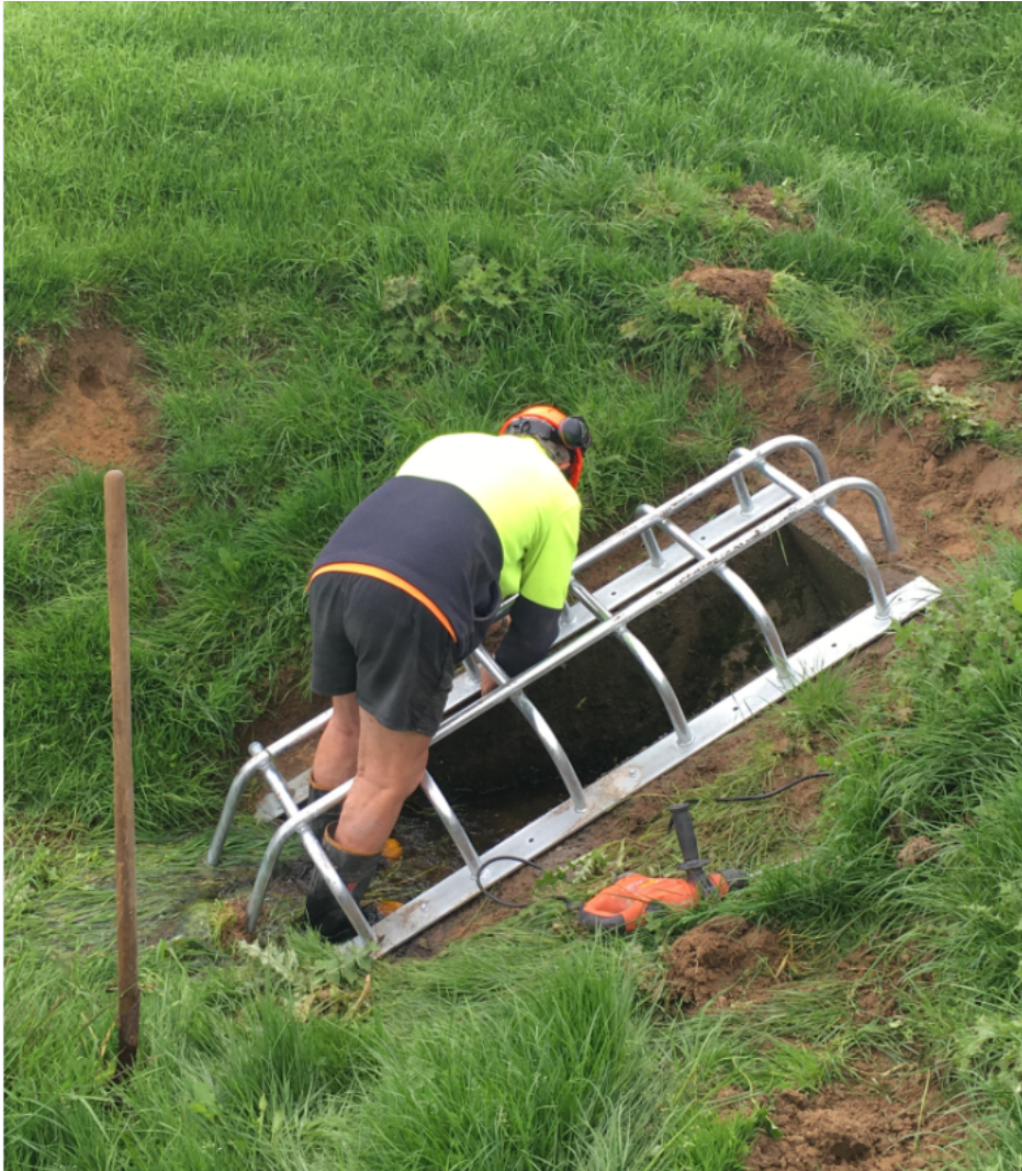
Inlet screen being replaced at dam 82
