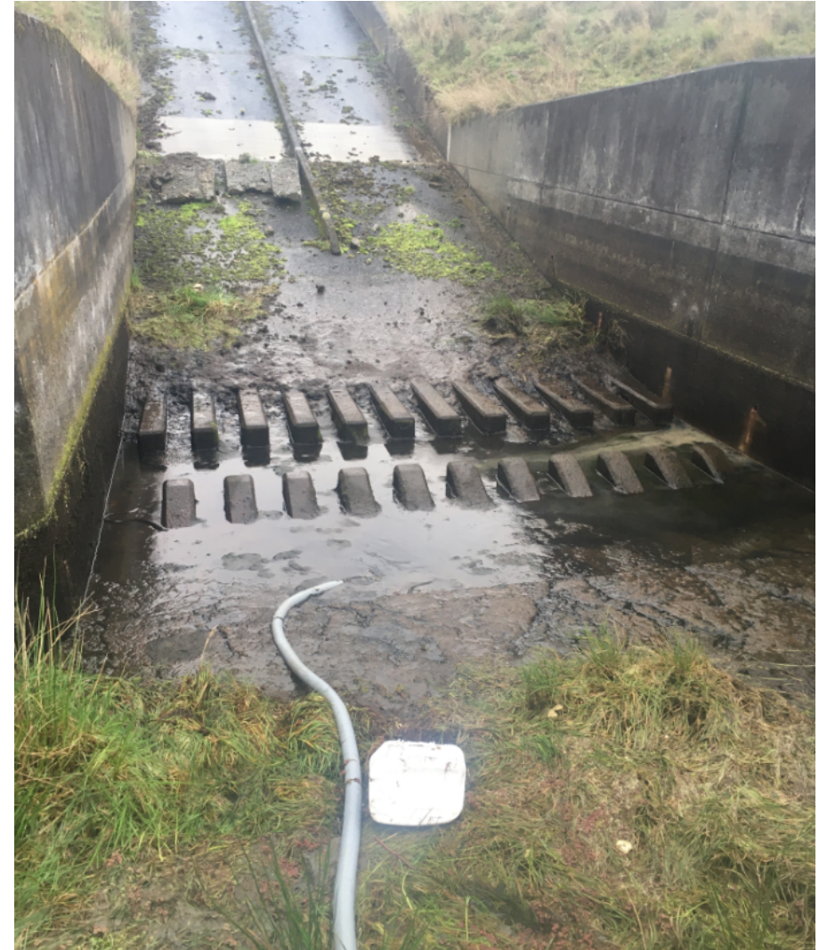
Dam 46 spillway pumped out to inspect dissipation blocks as recommended in Stantec review
