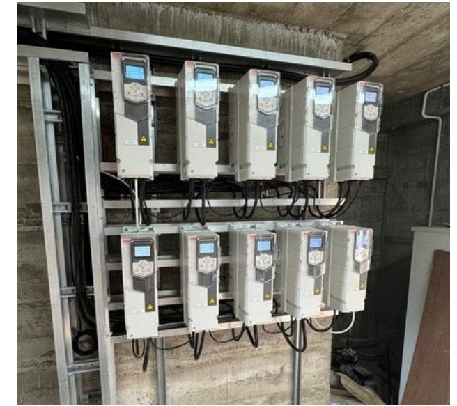
Newly installed variable speed drives for gate motor control
