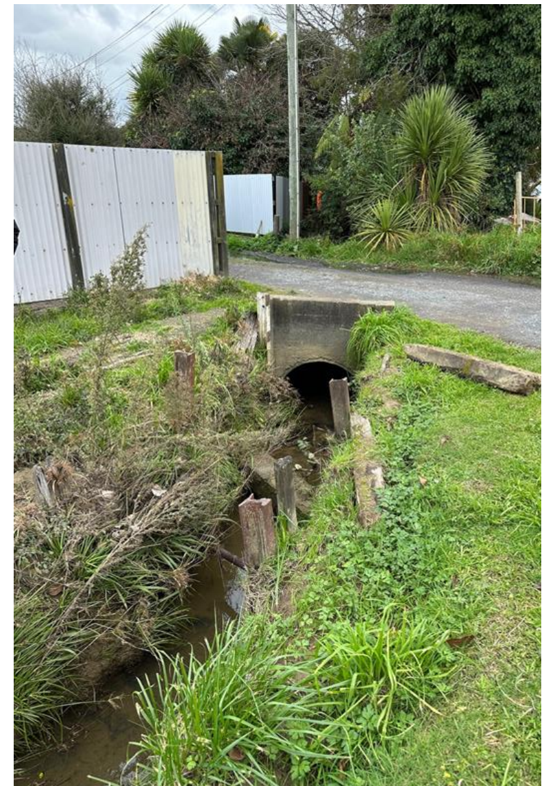
Culvert/ crossing a restriction point. Note there is at least one other vehicle crossing point.
