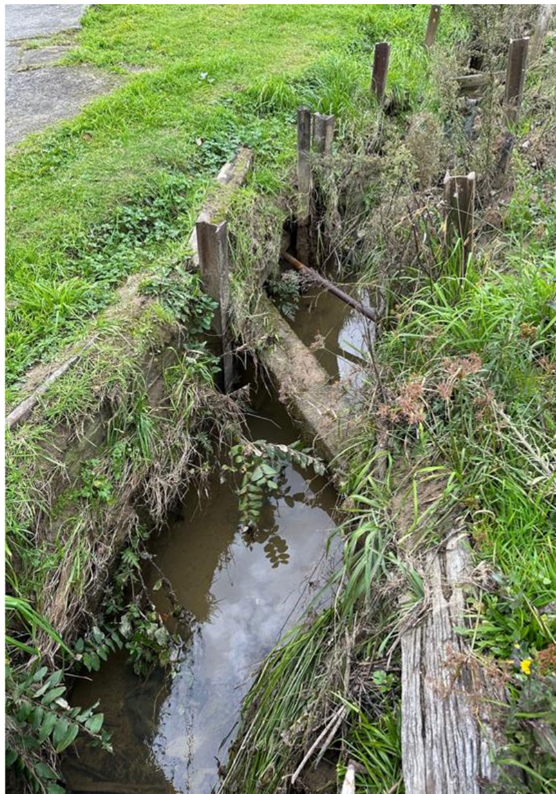
Channel between houses near the culvert/ crossing shown on right. Note a sewer pipe crosses the drain in this location.
