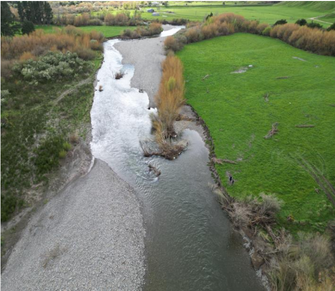
Mahoney's Farm tied-tree work. Pole planting and channel widening.
