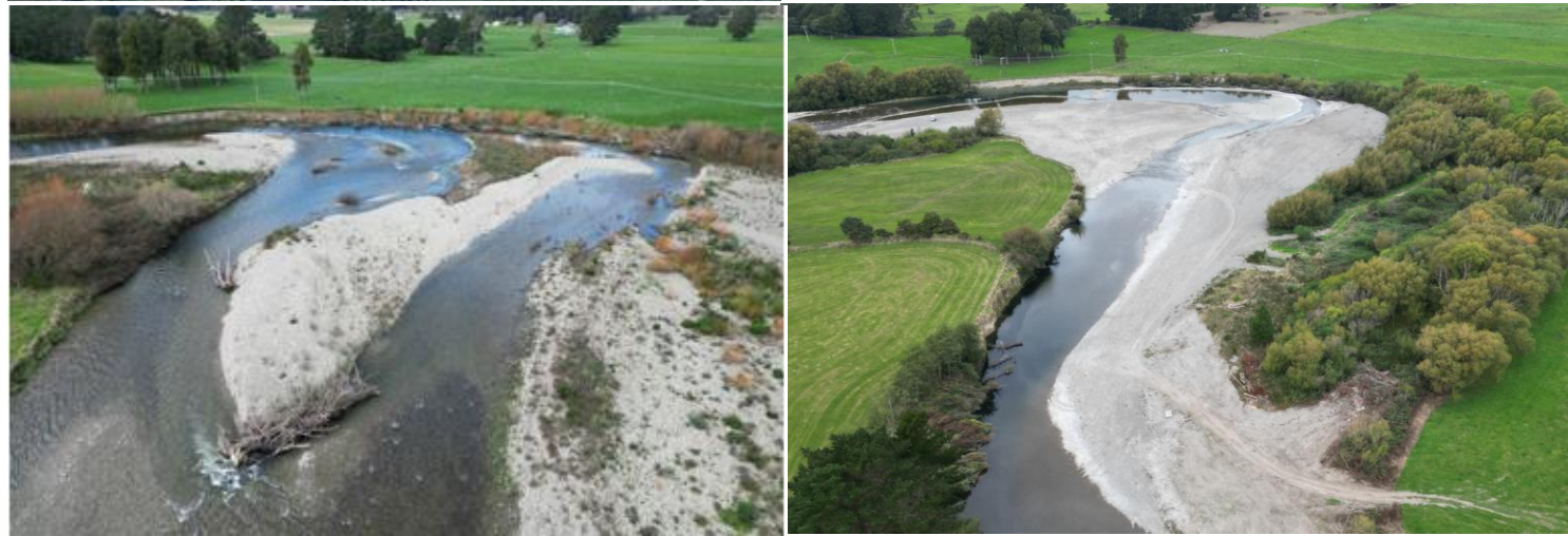
Example of beach pull back and ripping – Thurlows bend.
