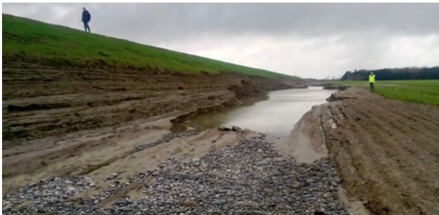
Figure 8: Inspection of a stopbank damaged during a storm event. Climate change is likely to increase the amount of asset inspection and repair work required.
