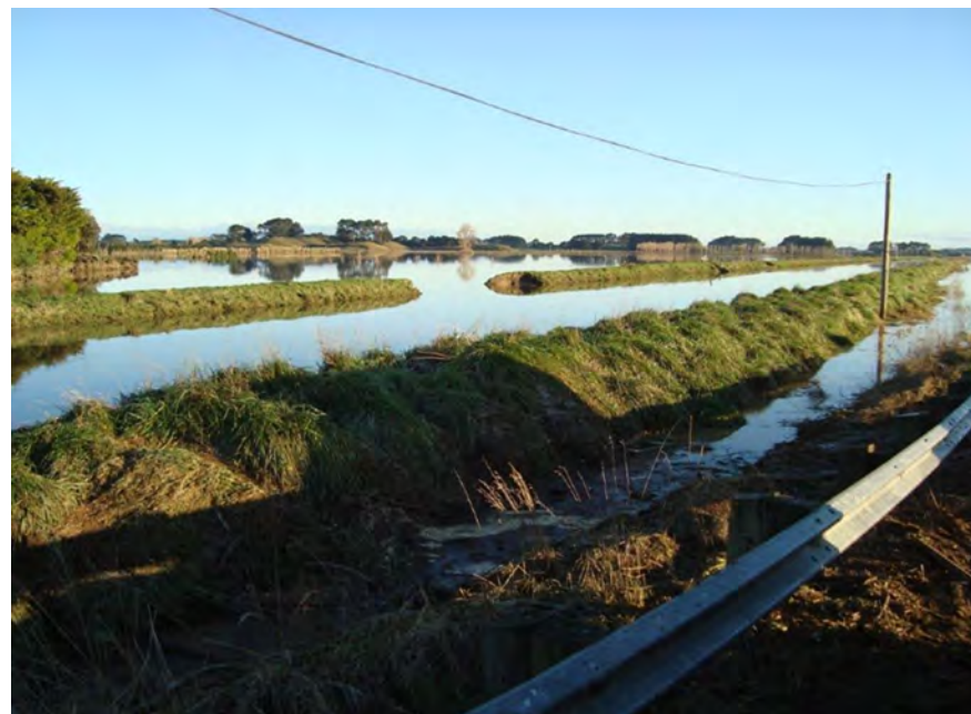
Figure 19: Example of asset failure. Stopbank breach in Sluggish Main Drain in the Te Kawai Drainage Scheme during the 2015 flood event.
