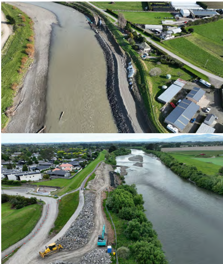
Figure 12: Photos in two flood protection upgrades completed as part of the Climate Resilience work programme. Above: rock armouring at Te Matai Road, Manawatu River. Below: Albert Street, Palmerston North.
