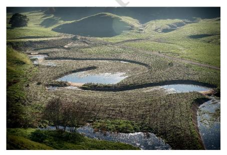
Figure 1: Newly constructed treatment wetland with weirs and spillways to slow down the flow of water and prevent depths greater than 500mm. 2
