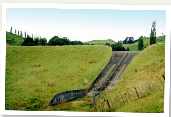
A spillway on a large dam
