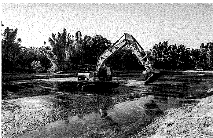
Picture 2: Removing biosolids from a sewage treatment pond.
